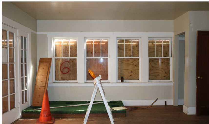
Looking north east inside the entry.
