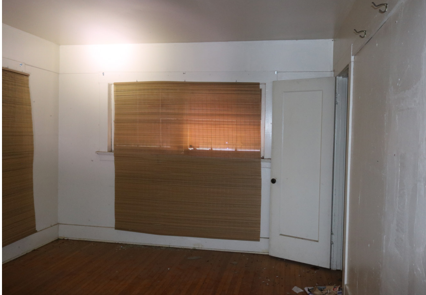
View looking south inside bedroom/ office at end of east wing.
