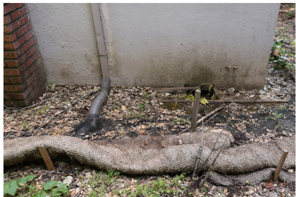
Coir rolls along west elevation (ARG, 2019).
