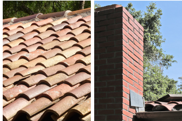
Clay tile roof (left); metal flashing at west chimney (right); (ARG, 2019).
