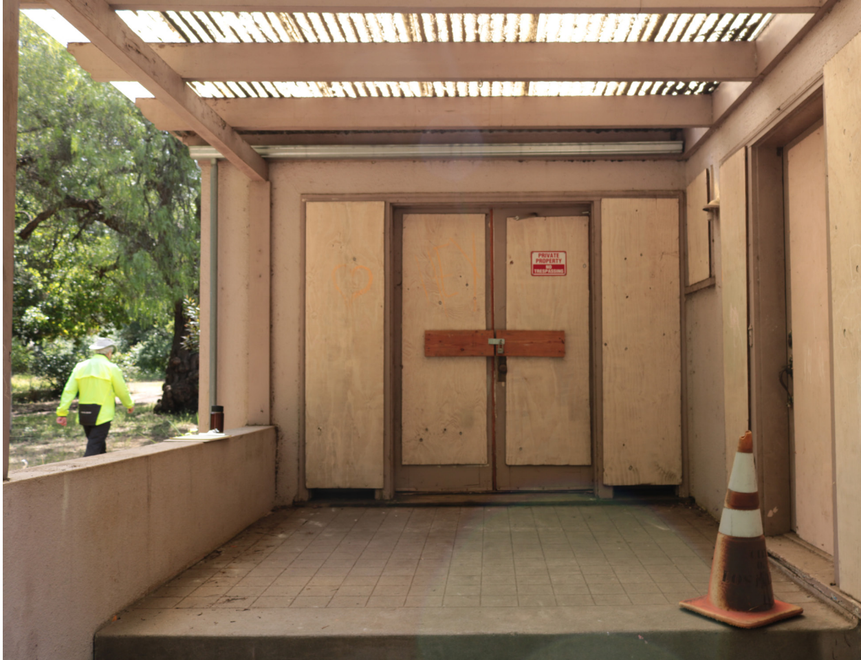
Main entrance to Halsey House, at northeast corner of building.
