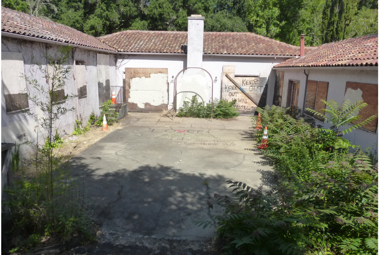
View looking north into enclosed courtyard.
