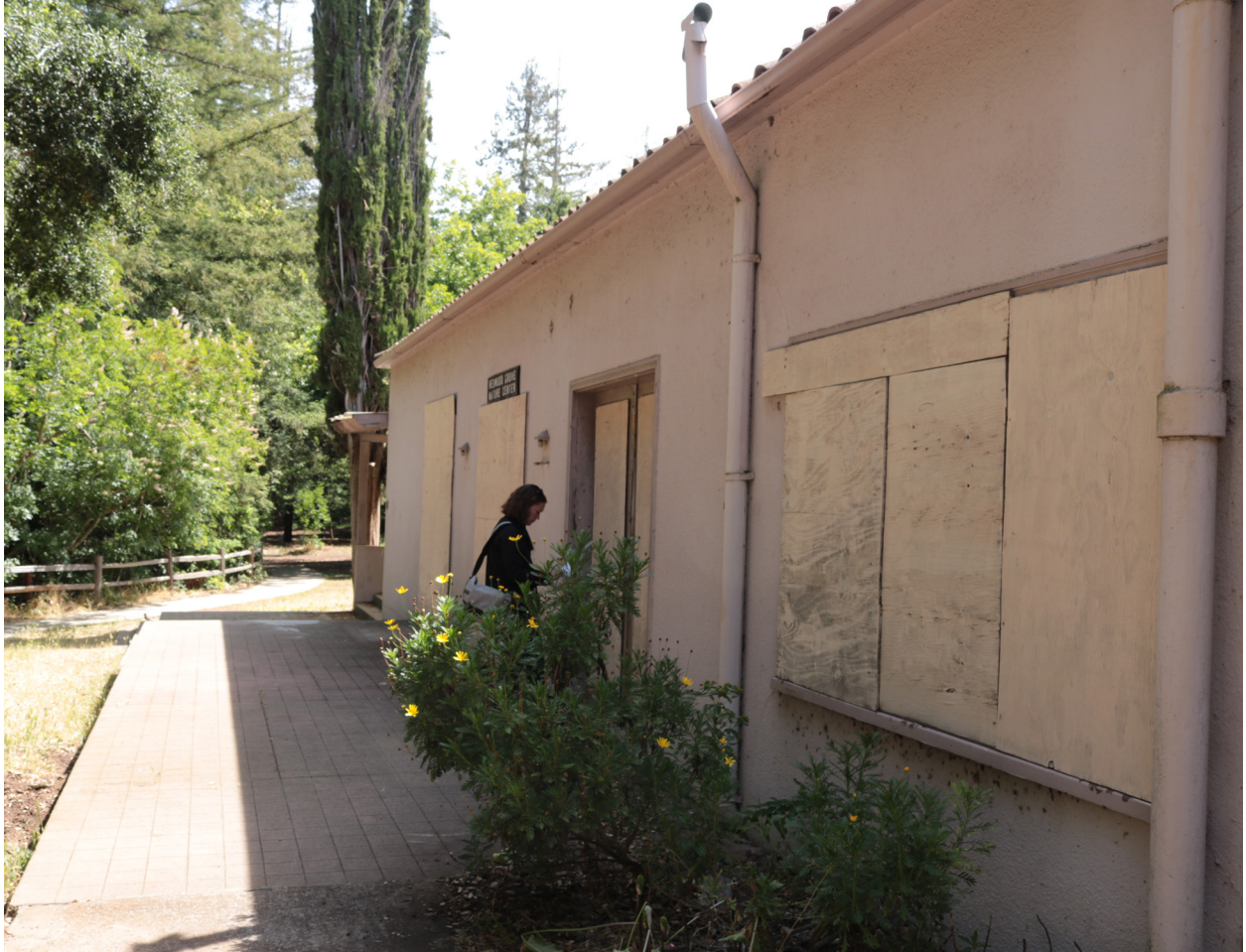
View of north elevation looking east.
