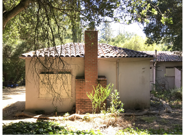
Photo #2 - West Elevation of the Northwest Appendage of the Building
