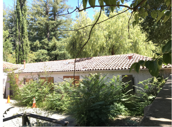
Photo #8 - West Elevation of the East Wing of the Building
