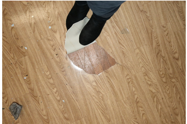
Original wood floor beneath sheet vinyl in the Animal Room (ARG, 2019).
