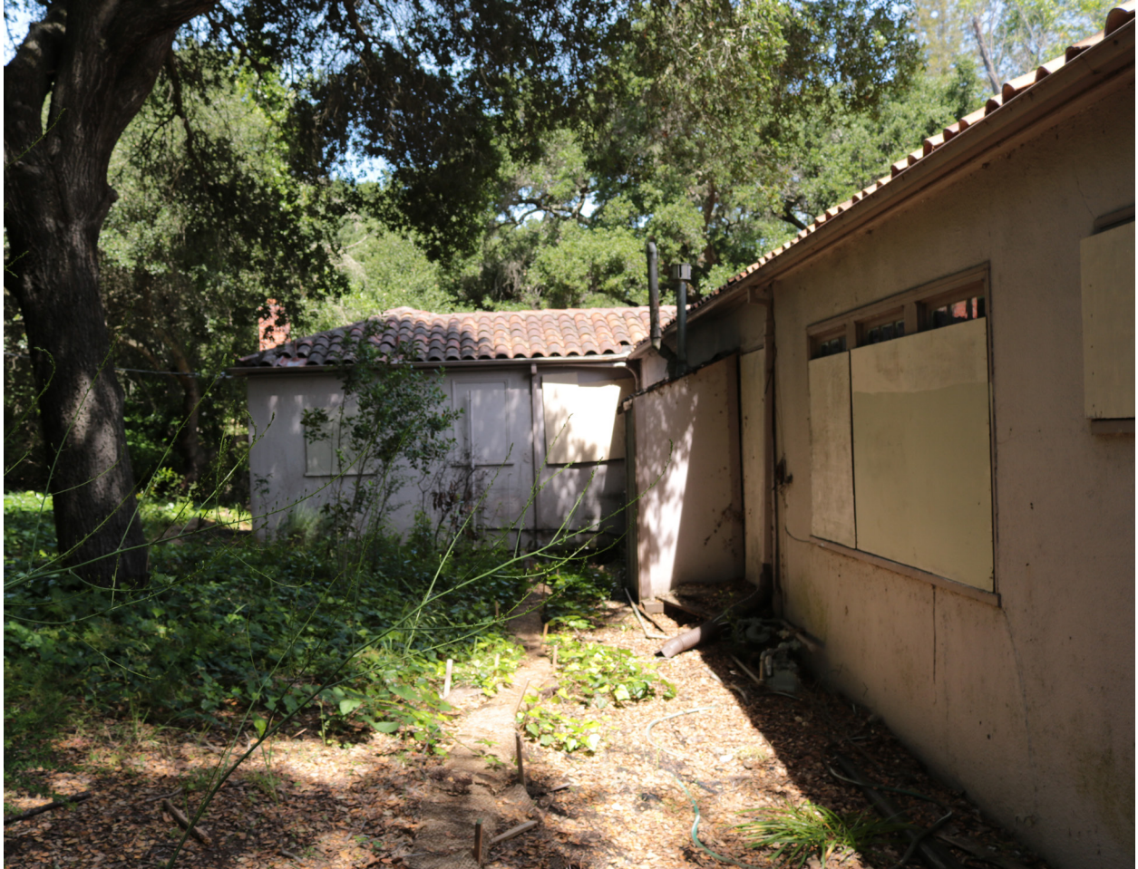
Looking north along the west elevation.
