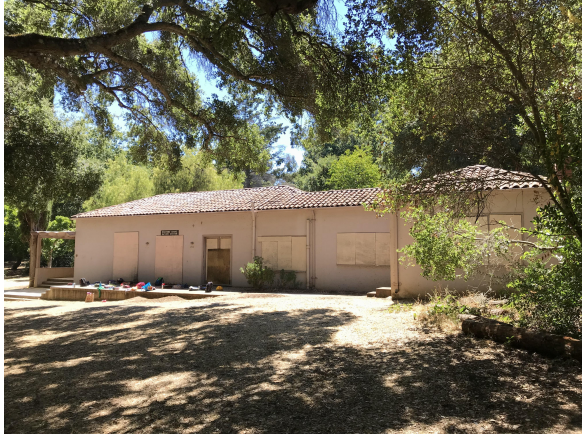
Photo #1 - North Elevation of the Building
