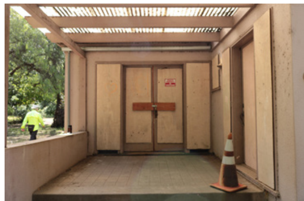
Figure 3. Primary entry porch (photo: ARG, May 2019).
