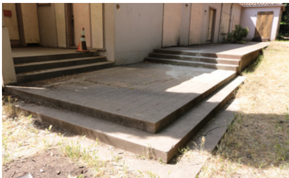
Figure 4. Concrete porch and terrace (photo: ARG, May 2019).
