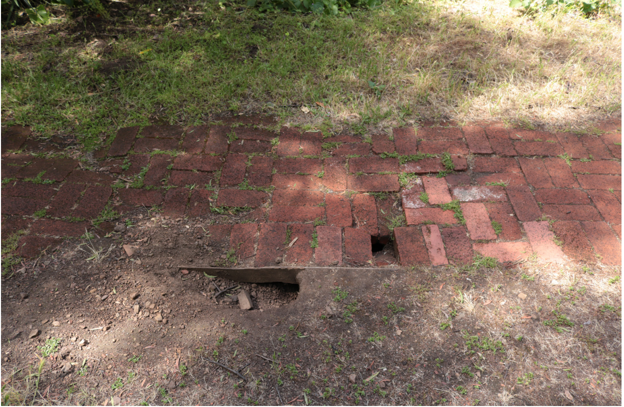
View of walkway paving along east elevation.
