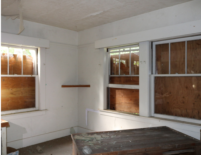
View looking south inside Discovery Lab.
