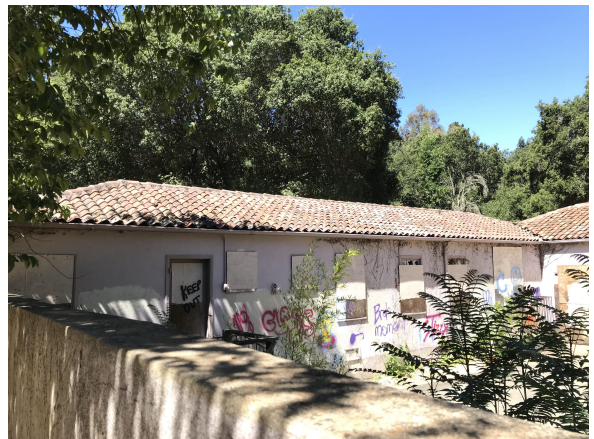
Photo #6 - East Elevation of the West Wing of the Building
