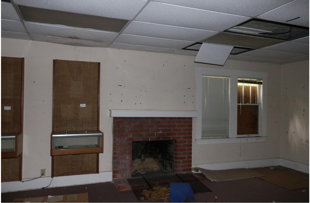
Overall view inside Ohlone room.
