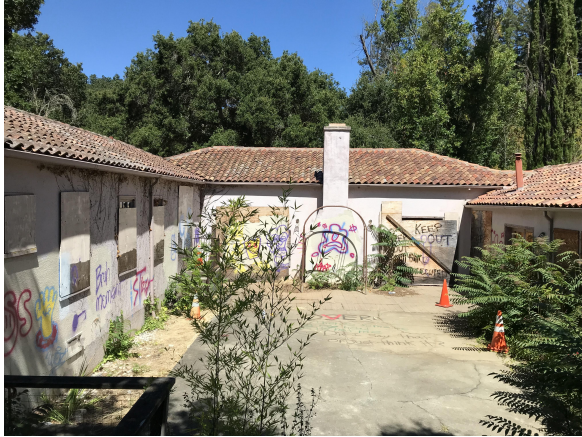
Photo #7 - South Elevation of the North Wing of the Building
