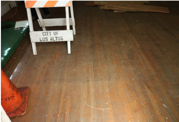
Original wood flooring in the Entry (ARG, 2019).
