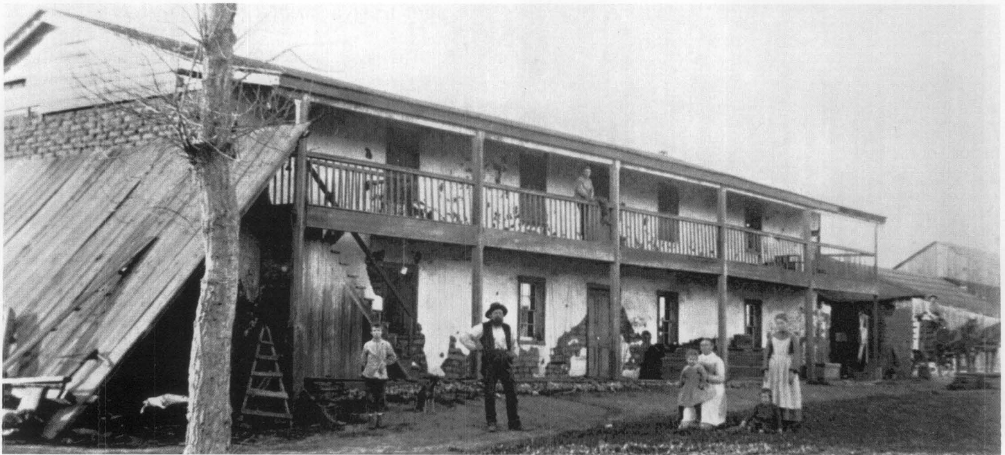
Figure 6. Historical photographs are an invaluable aid and time saver in establishing a building's original construction and evolution; in guiding the replication of missing features; and even in understanding existing material deterioration. The availability of information, such as archival photographs, surviving original architectural drawings, or HABS documentation, has a direct bearing on the cost of preparing a historic structure report. In this circa 1890 photo of the Rancho San Andrés Castro Adobe, the "lumbering up" on the south end is a character-defining feature of adobe construction, rarely seen today. Photo: Historic photograph from the Historic Structure Report for Rancho San Andrés Adobe by Edna Kimbro, State Historian, California State Parks, Monterey District.
