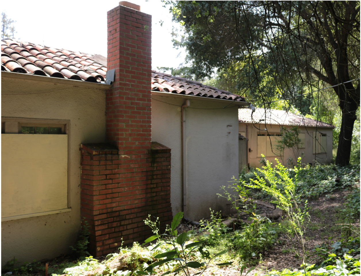
Looking south along the west elevation.
