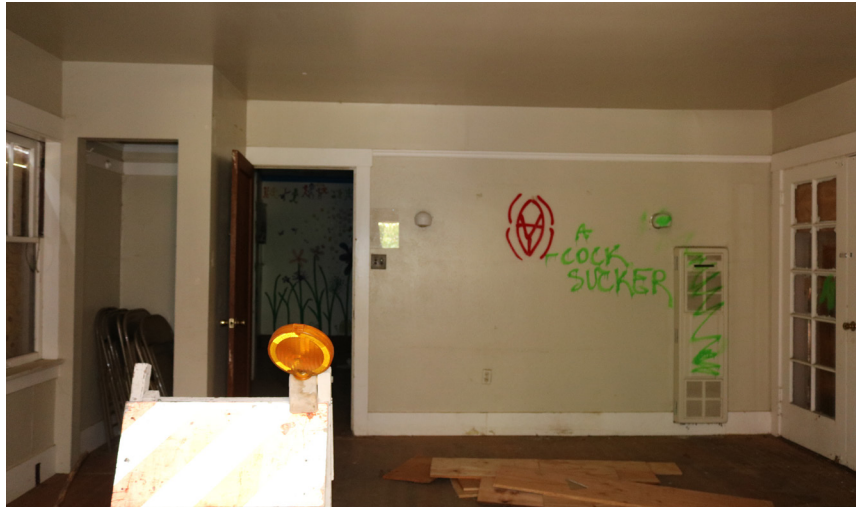
View looking south inside main entrance.
