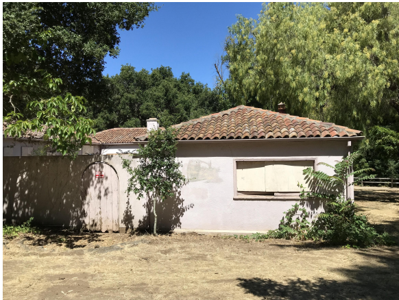
Photo #9 - South Elevation of the East Wing of the Building
