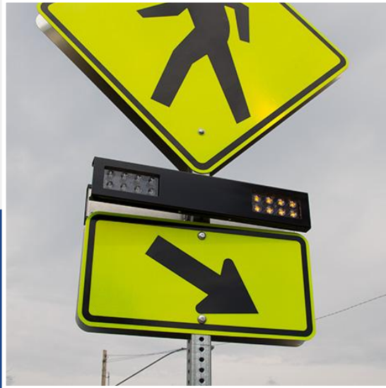
Rectangular Rapid Flashing Beacon (disapproved by FHWA)
