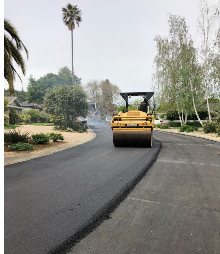
1.5-inch thick Asphalt Overlay
