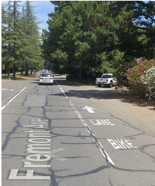
Existing Bike Lane
