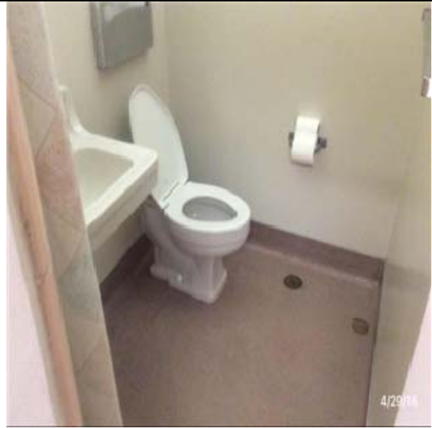
D2013 Lavatories:- View of Wall Hung Lavatories
