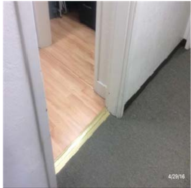
C1011 Fixed Partitions:- View of Wood framing with board finish
