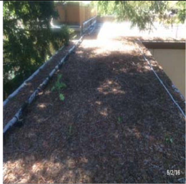
B3011 Roof Finishes:- View of BUR (Built-up Roofing) Covering to Canopy
