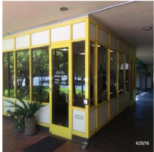
B2023 Storefronts:- View of Storefronts - Glazed Aluminum Framed with Swing Doors
