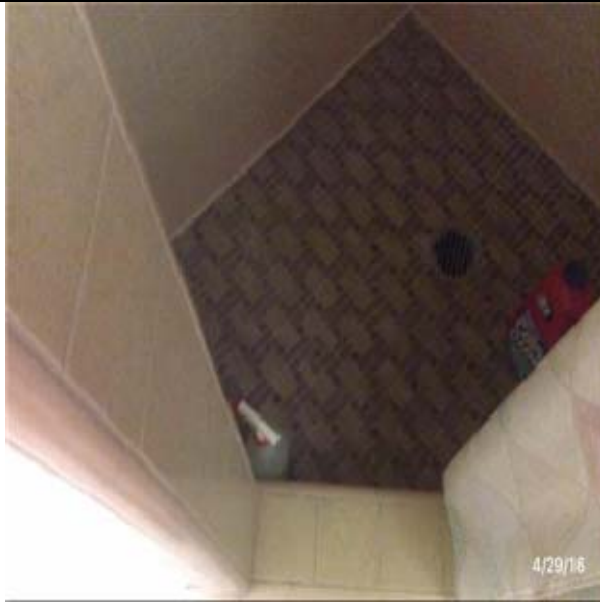
C3024 Flooring:- View of Ceramic Tile
