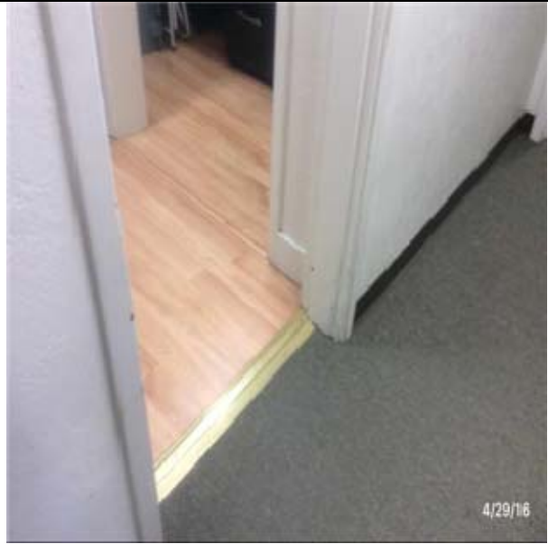
C3024 Flooring:- View of Laminate Wood Floors
