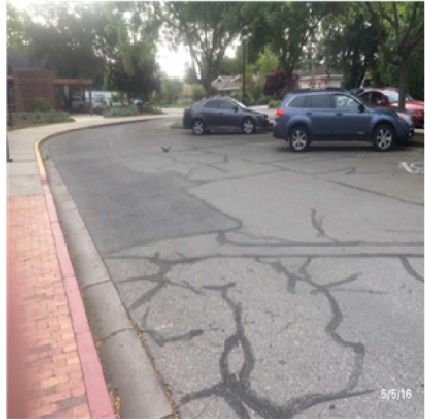
G2021 Bases and Sub-Bases:- View of Seal Coating including Re-Striping
