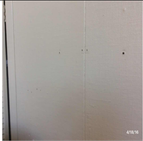
C1011 Fixed Partitions:- View of GWB Stud Walls
