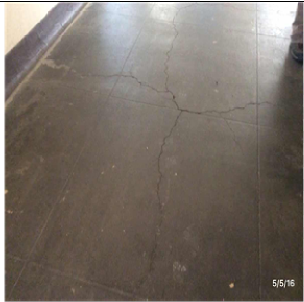
G2031 Paving & Surfacing:- View of Concrete Paving
