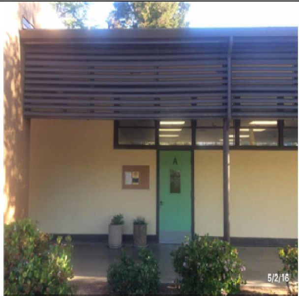
B2014 Exterior Sun Control Devices:- View of Exterior Sun Control Louvers
