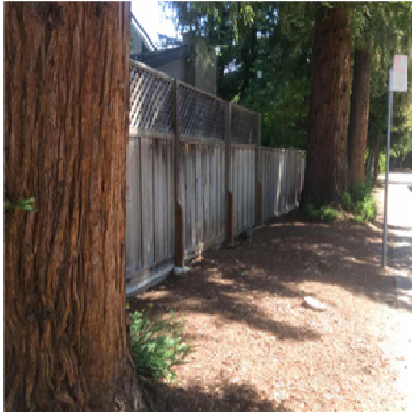
G2041 Fences & Gates:- View of Wood Fence
