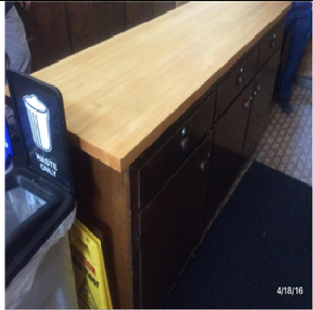
E1095 Unit Kitchens:- View of Unit Kitchens - Counter Top - Wood
