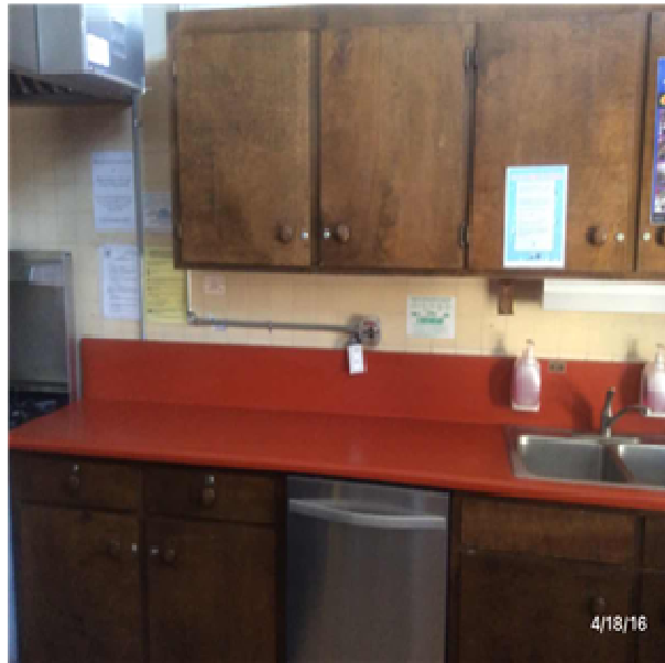
E2012 Fixed Casework:- View of Fixed Casework - Wall Mounted Cabinets - Standard
