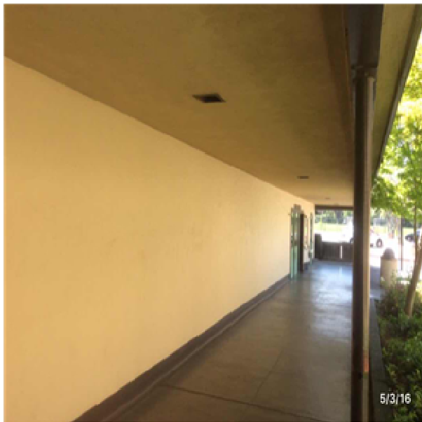
B2016 Exterior Soffits:- View of Exterior Soffits
