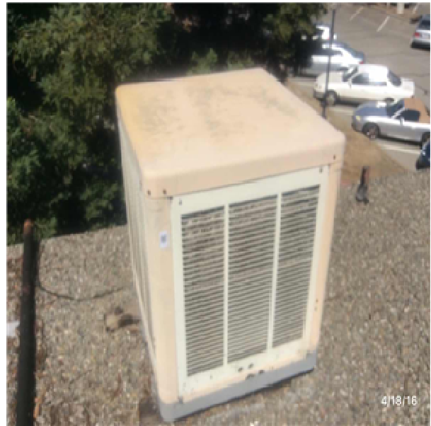
D3051 Terminal Self-Contained Units:- View of Evaporative Cooler Unit (Medium)
