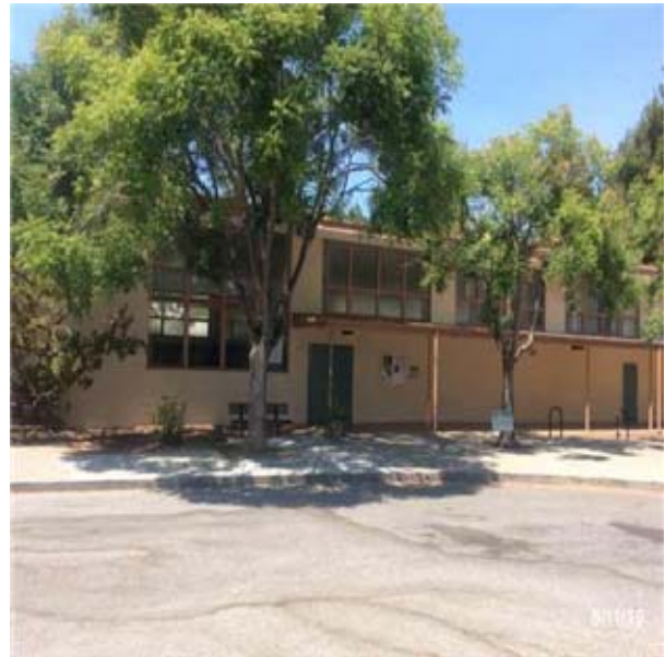
B2032 Solid Exterior Doors:- View of Double Solid Core Wood Doors
