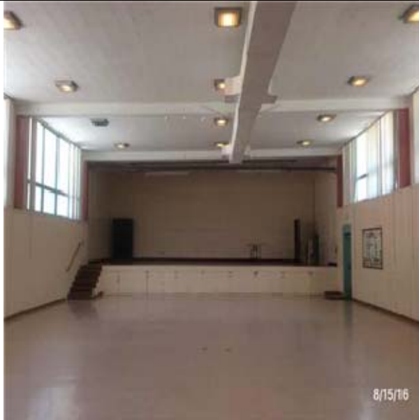
B1012 Upper Floors Construction:- View of Wood Beams and Joist Supporting Timber Decking
