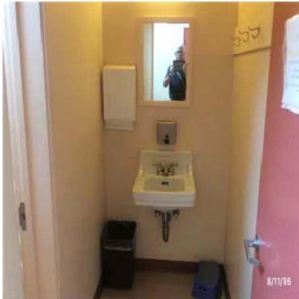
D2013 Lavatories:- View of Wall Hung Lavatories
