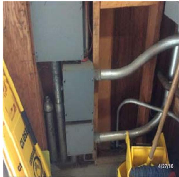
B1033 Wood Frame Structure:- View of Structural Wood Columns and Beams
