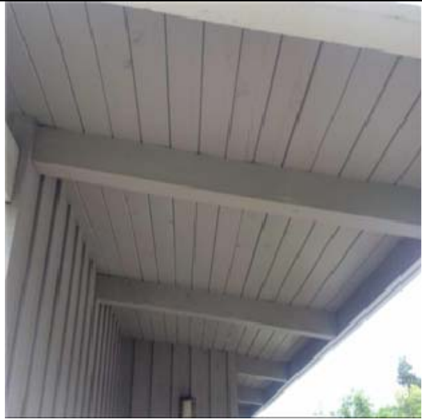
B2016 Exterior Soffits:- View of Exterior Soffits
