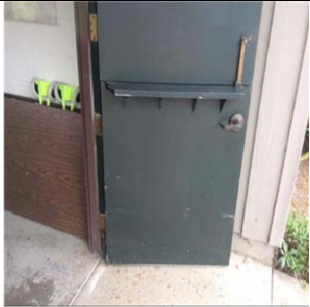
B2039 Other Doors & Entrances:- View of Exterior Single HM Doors
