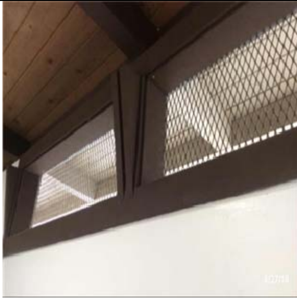
B2013 Exterior Louvers, Screens, and Fencing:- View of Metal screens in wood frames
