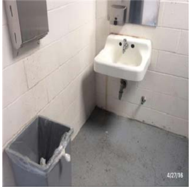
D2013 Lavatories:- View of Wall Hung Lavatories
