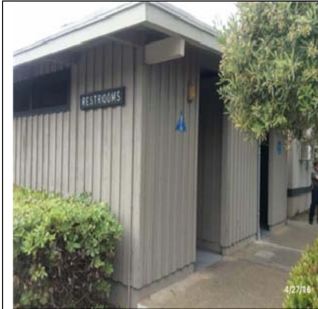
A1011 Wall Foundations:- View of Slab-on-Grade Reinforced Concrete Raft
