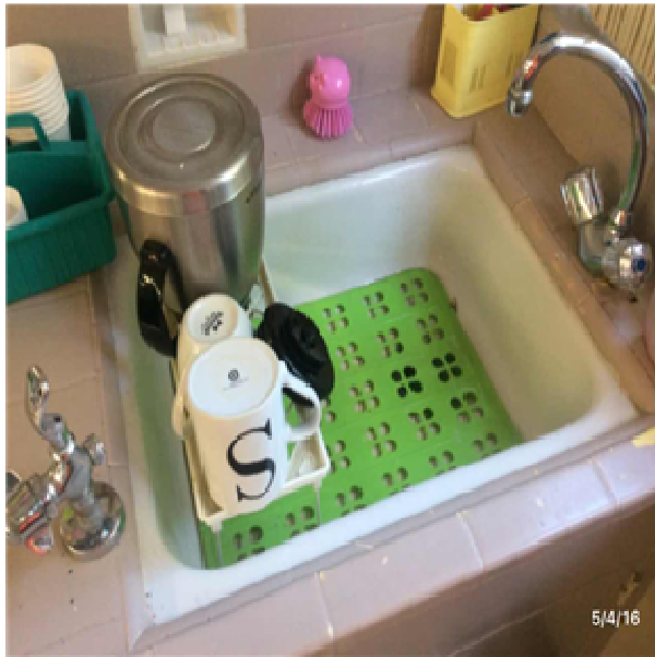
D2013 Lavatories:- View of Vanity Top Lavatories
