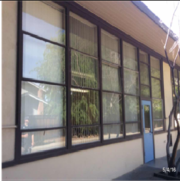
B2021 Windows:- View of Steel Window Units - Casement, Double Hung, Vent or Sliding
