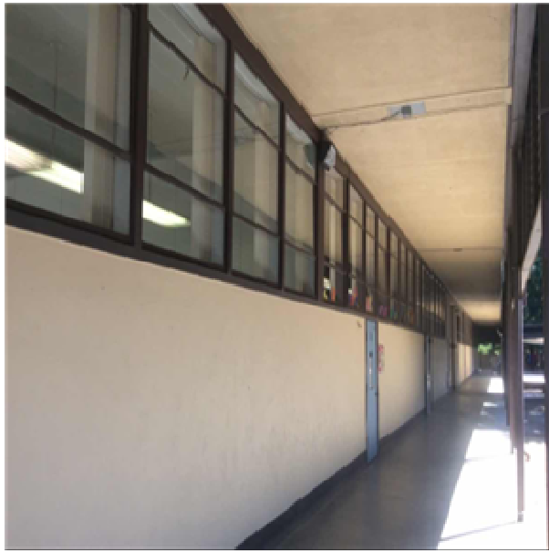
B2016 Exterior Soffits:- View of Exterior Soffits
