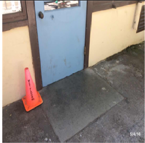
B2032 Solid Exterior Doors:- View of Single Solid Core Wood Doors
