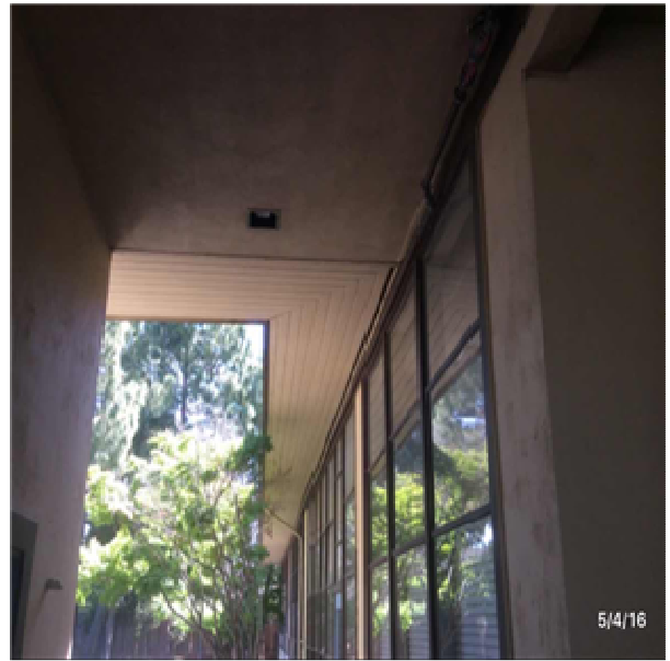
B2016 Exterior Soffits:- View of Exterior Soffits
