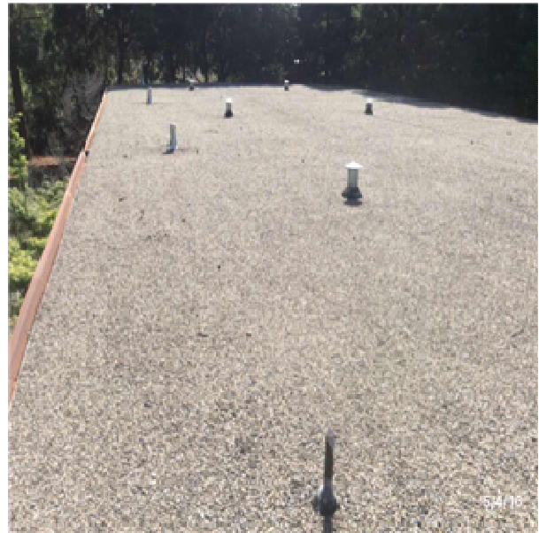
B3011 Roof Finishes:- View of BUR (Built-up Roofing) System
