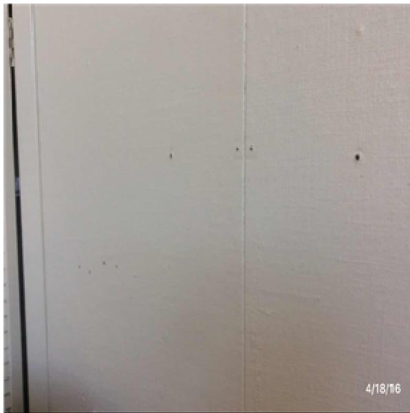
C1011 Fixed Partitions:- View of Stud Walls with board finish
