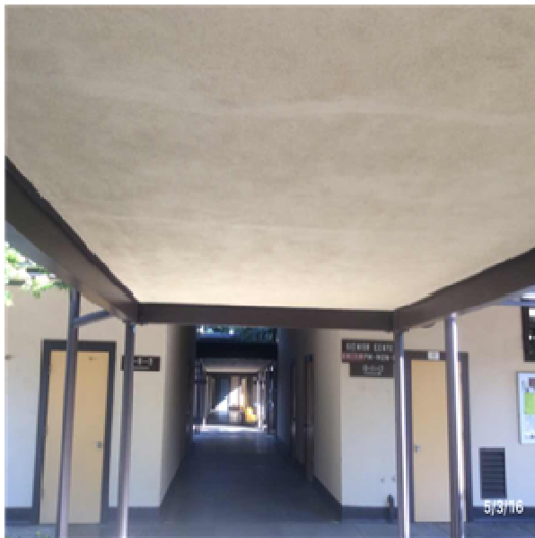
B2016 Exterior Soffits:- View of Exterior Soffits to Canopy
