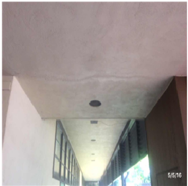
B2016 Exterior Soffits:- View of Exterior Soffits to Corridor
