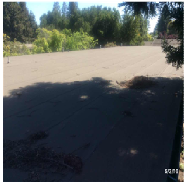
B3011 Roof Finishes:- View of BUR (Built-up Roofing) Covering
