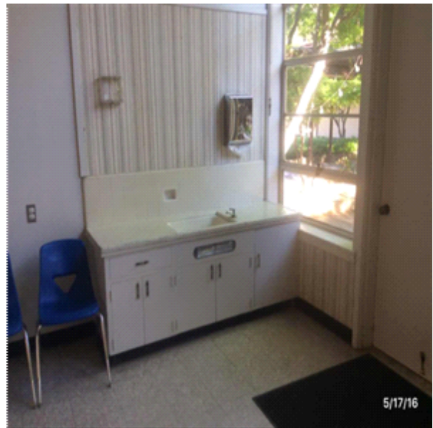
E1095 Unit Kitchens:- View of Unit Kitchens - Counter Top - Ceramic
