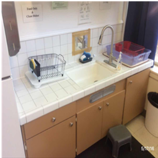
E2012 Fixed Casework:- View of Kitchen Cabinet(s) - Standard
