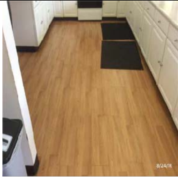
C3024 Flooring:- View of Laminate Wood Floors
