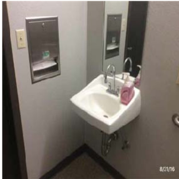
D2013 Lavatories:- View of Wall Hung Lavatories
