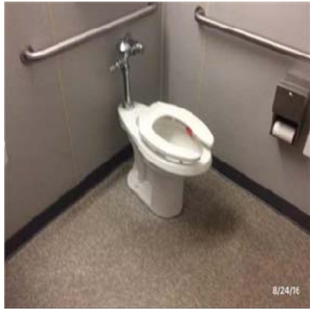
C3024 Flooring:- View of Vinyl Sheet
