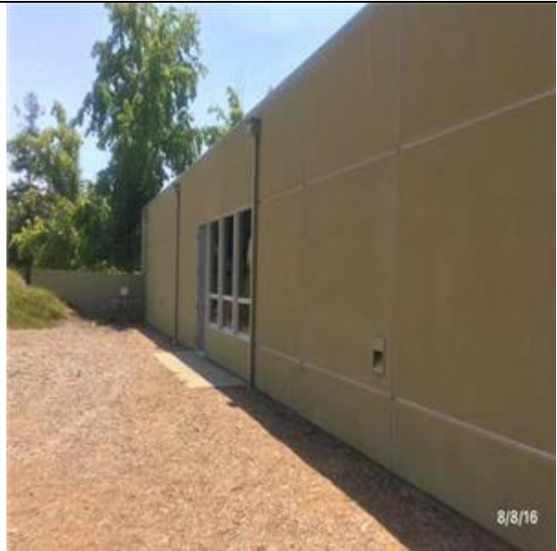
B2011 Exterior Wall Construction:- View of EIFS (Synthetic Stucco) Wall Panels - Standard
