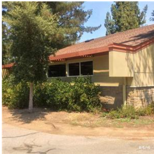
B2012 Parapets:- View of Metal Capping
