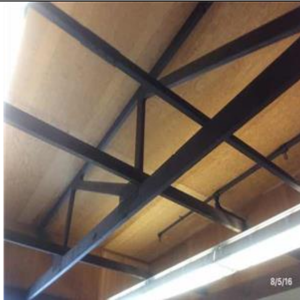
B1022 Pitched Roof Construction:- View of Manufactured Wood Trusses
