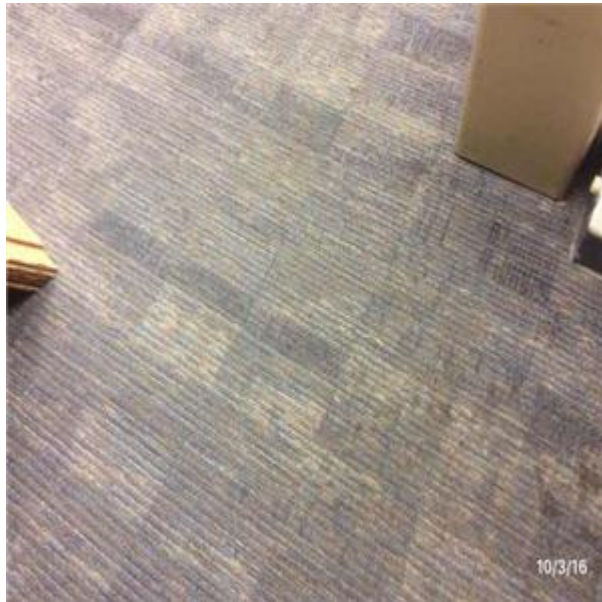
C3025 Carpeting:- View of Carpet Tiles – Standard
