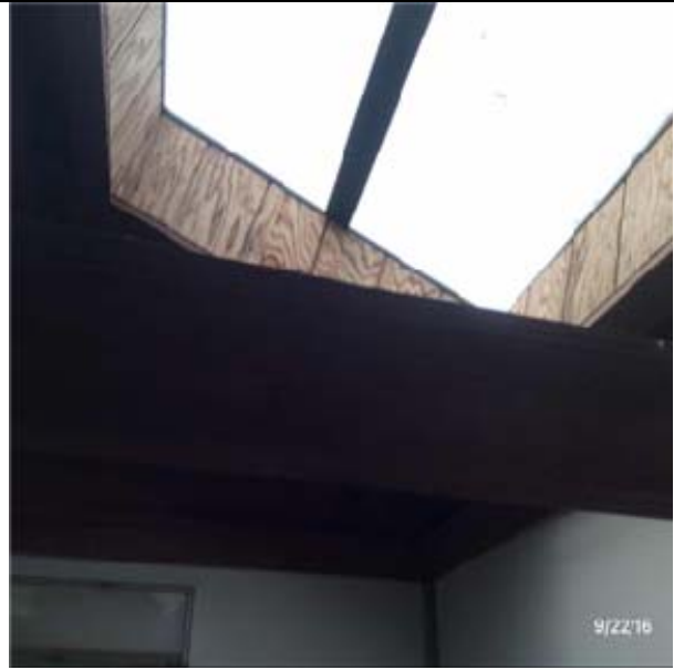
B3021 Glazed Roof Openings:- View of Skylight – Plastic
