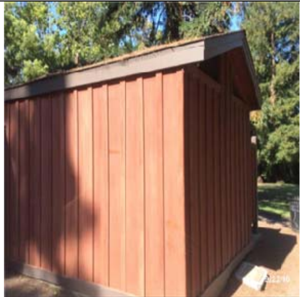
B2011 Exterior Wall Construction:- View of Wood Board and Batten Cladding
