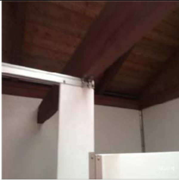
C3031 Ceiling Finishes:- View of Wood Ceiling (Stained)
