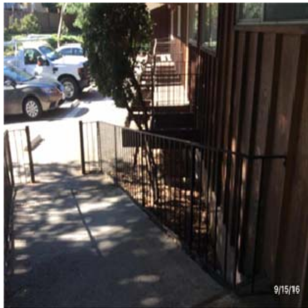
B1014 Ramp(s):- View of Ramp(s) - Steel Construction
