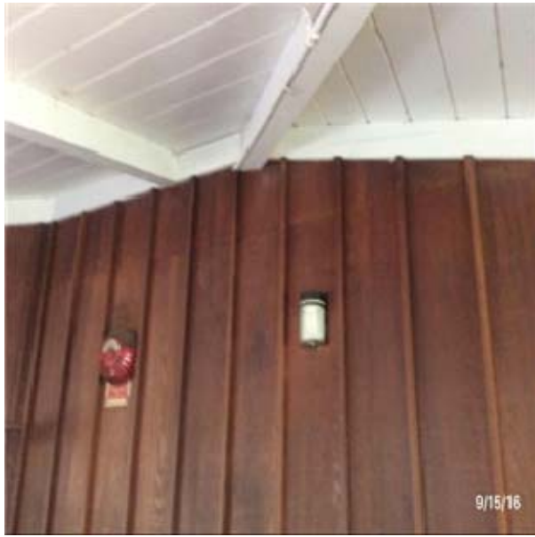
B2011 Exterior Wall Construction:- View of Wood board and batten
