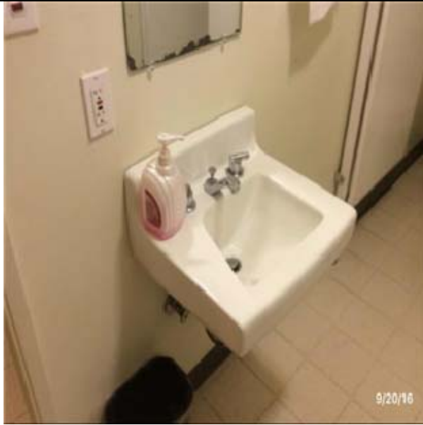
D2013 Lavatories:- View of Wall Hung Lavatories
