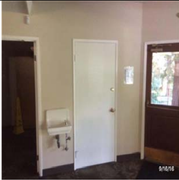
C1021 Interior Doors:- View of Single Solid Core Wood Doors
