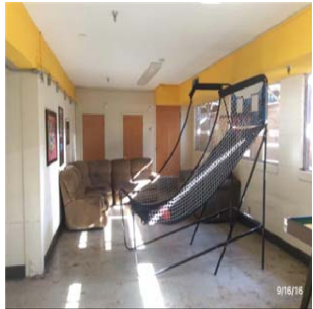
C3023 Hardeners and Sealers:- View of Seal Floor Coating
