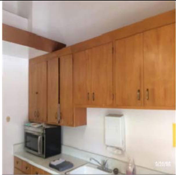
E1095 Unit Kitchens:- View of Unit Kitchens - Wall Mounted Cabinets - Standard
