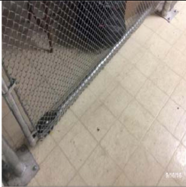
C3024 Flooring:- View of Vinyl Sheet
