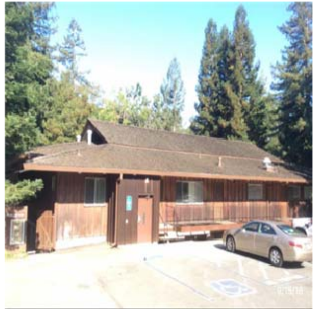
B3011 Roof Finishes:- View of Wood Shingle Roof
