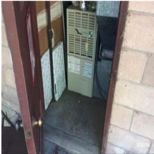
B2039 Other Doors & Entrances:- View of Single Wood Louvered Doors
