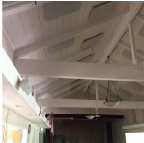
C3031 Ceiling Finishes:- View of Wood Ceiling – Painted or Stained
