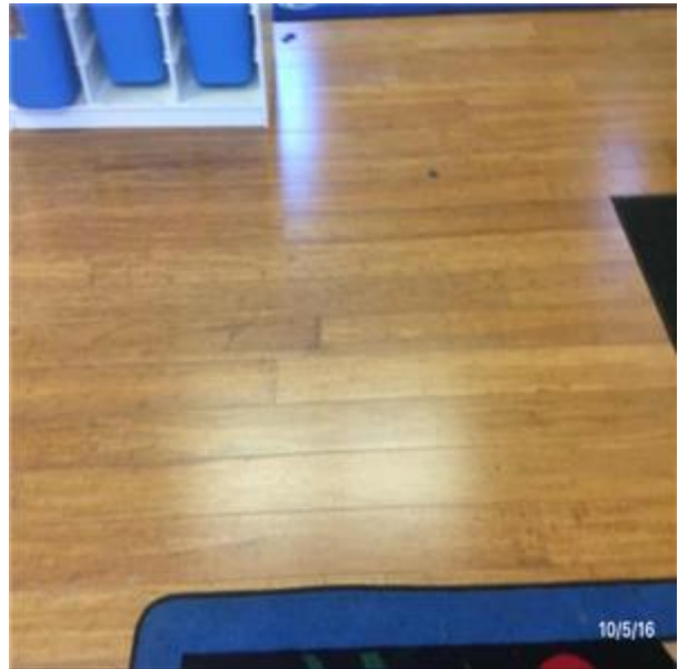
C3024 Flooring:- View of Wood Flooring – Redwood
