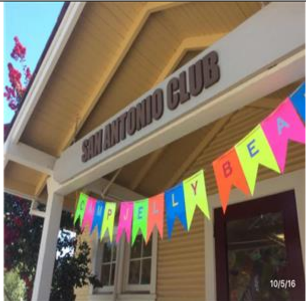
B1023 Canopies:- View of Canopies - Wood Joists Supporting Exterior Grade Plywood
