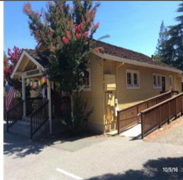
B1014 Ramp(s):- View of Ramp - Wood Construction
