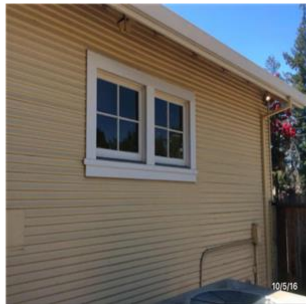
B2011 Exterior Wall Construction:- View of Wood Clapperboard Siding
