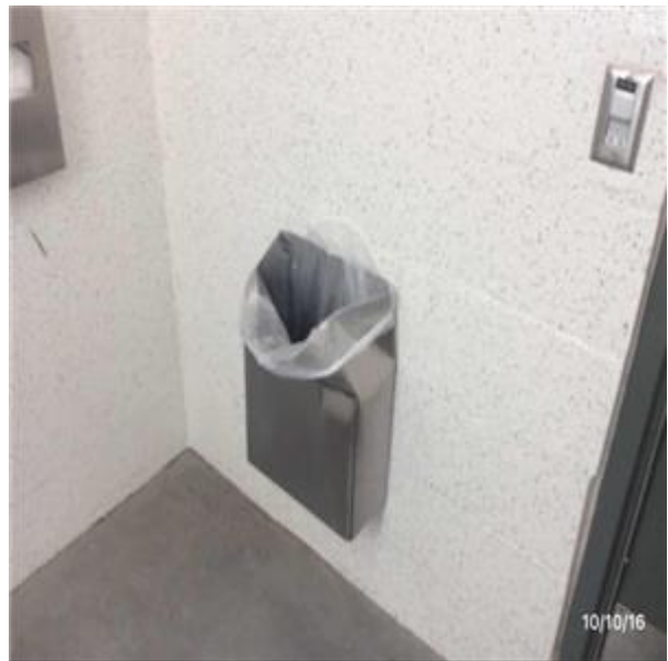
C1011 Fixed Partitions:- View of CMU Walls
