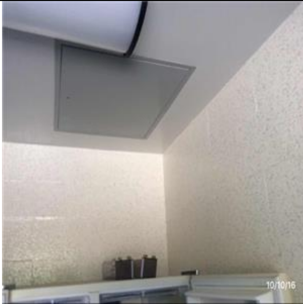
C3012 Wall Finishes to Interior Walls:- View of Painted Finish - Standard
