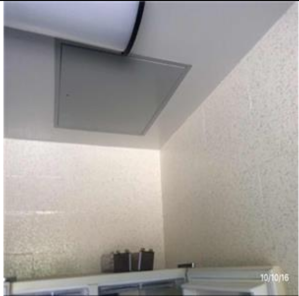
C3031 Ceiling Finishes:- View of GWB Ceiling
