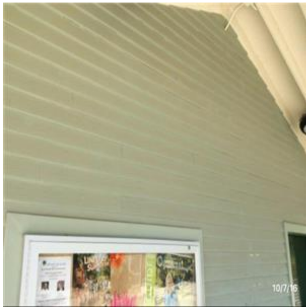
B2011 Exterior Wall Construction:- View of Cementitious Siding
