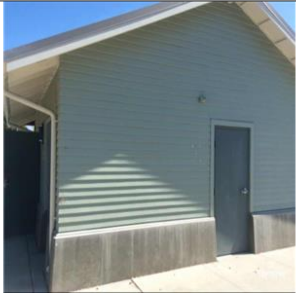
B2011 Exterior Wall Construction:- View of Cast-in-Place Concrete Walls
