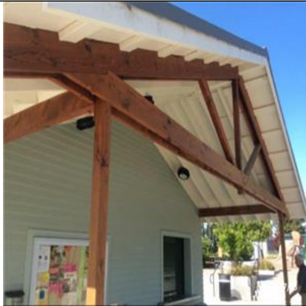
B1022 Pitched Roof Construction:- View of Traditional Wood Beams and Rafters
