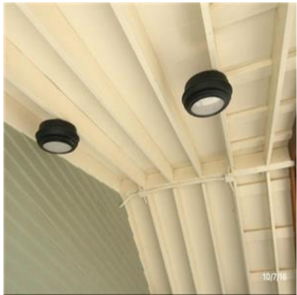
B2016 Exterior Soffits:- View of Exterior Soffits
