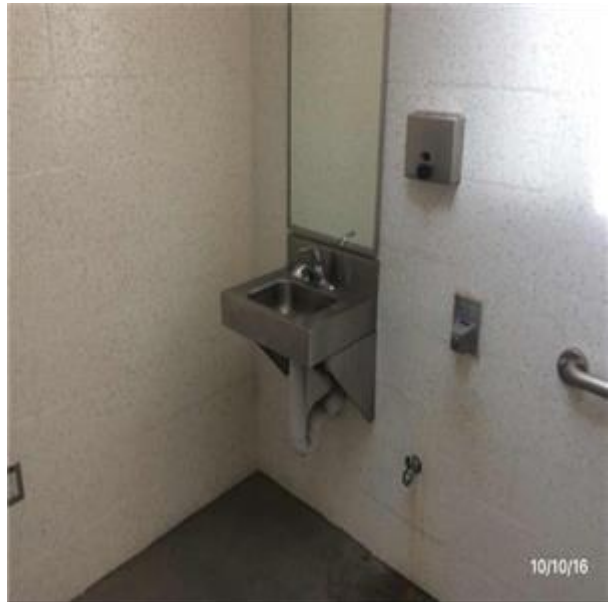
D2013 Lavatories:- View of Wall Hung Lavatories
