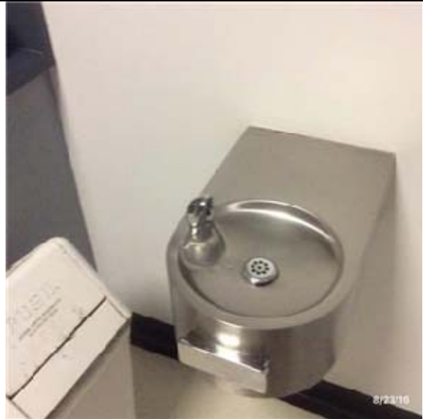
D2018 Drinking Fountains and Coolers:- View of Wall Mounted Standard Drinking Fountain (Single)
