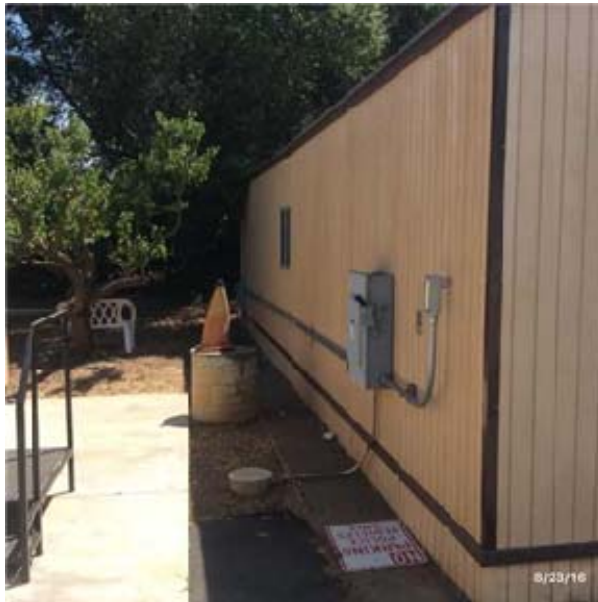
F1012 Pre-engineered Structures:- View of PreFab Modular Building #2
