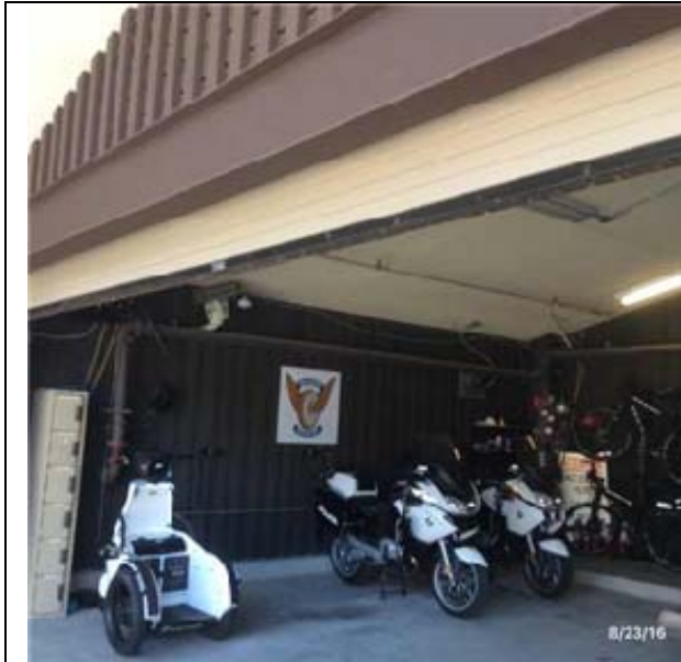
B1031 Steel Frame Structure:- View of Steel Frame Structure
