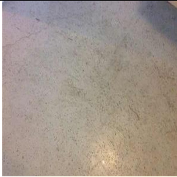
C3023 Hardeners and Sealers:- View of Epoxy Floor Coating
