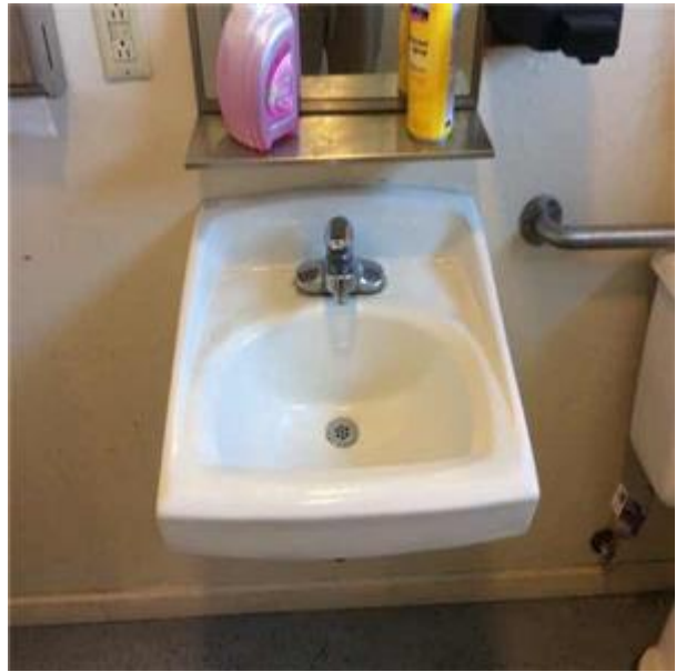
D2013 Lavatories:- View of Wall Hung Lavatories
