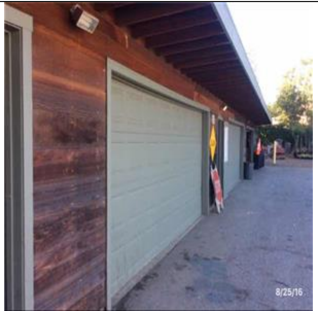
B2034 Overhead Doors:- View of Overhead Doors
