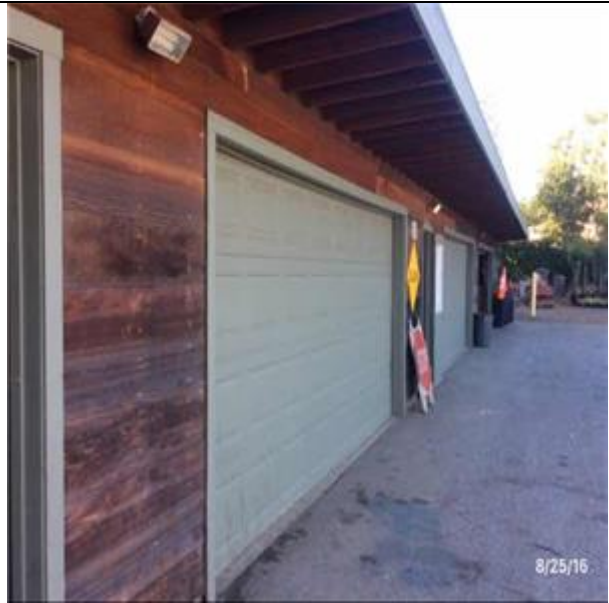
B1021 Flat Roof Construction:- View of Wood Decking
