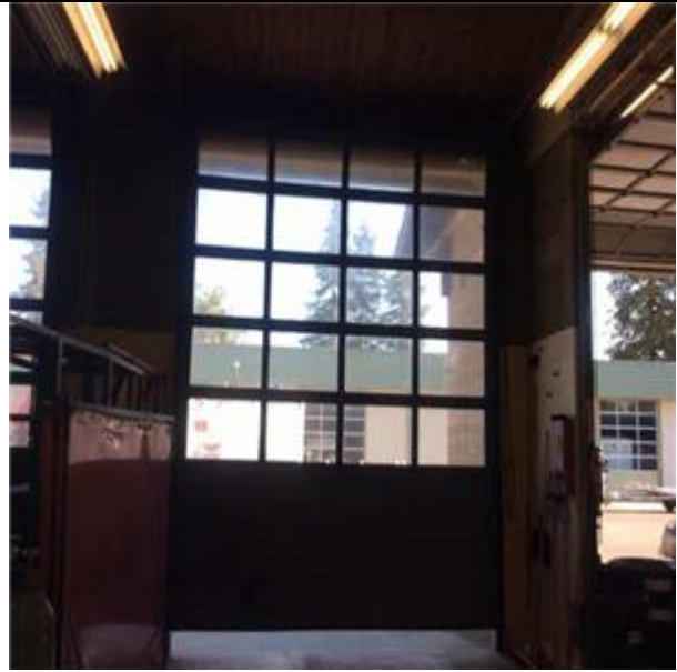
B2034 Overhead Doors:- View of Rolling Overhead Doors, Manual
