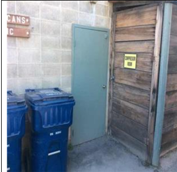
B2039 Other Doors & Entrances:- View of Single HM Doors
