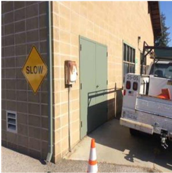
B2039 Other Doors & Entrances:- View of Double HM Doors
