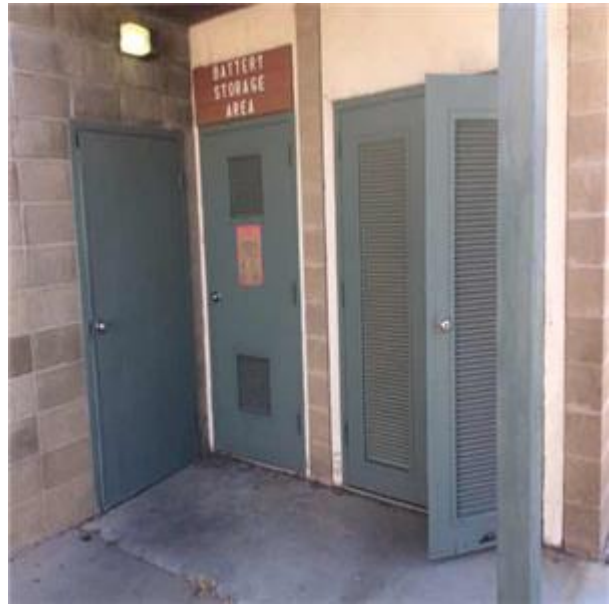
B2039 Other Doors & Entrances:- View of Double HM Louvered Doors
