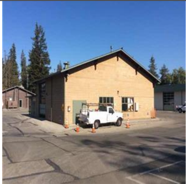
B2011 Exterior Wall Construction:- View of Exposed CMU Walls
