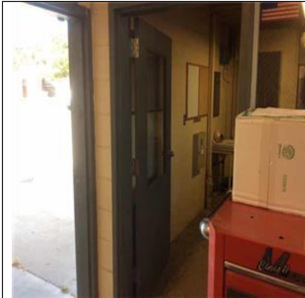
C1021 Interior Doors:- View of Interior Single Hollow Metal Door(s)
