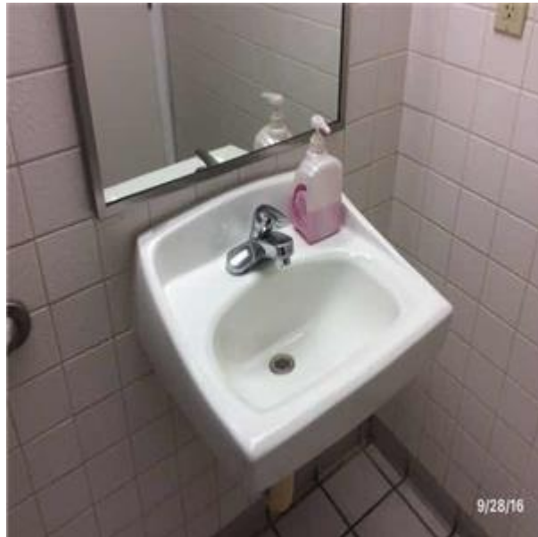
D2013 Lavatories:- View of Wall Hung Lavatories
