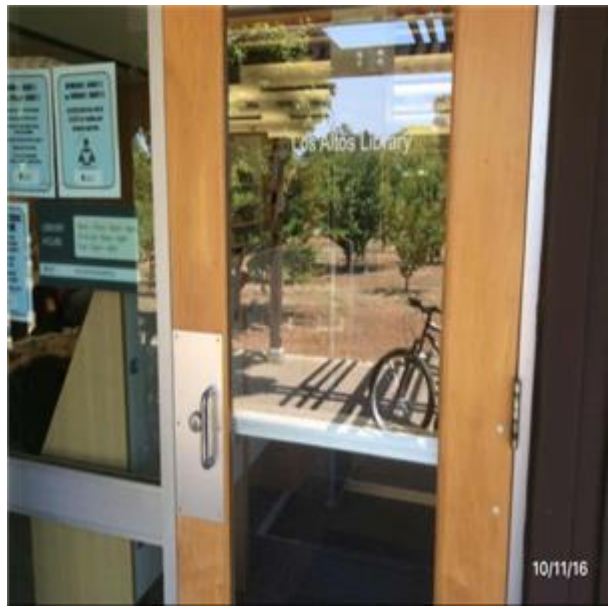
B2031 Glazed Doors & Entrances:- View of Single Wood Glazed Doors
