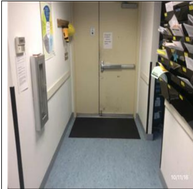
B2039 Other Doors & Entrances:- View of Single Hollow Metal Doors
