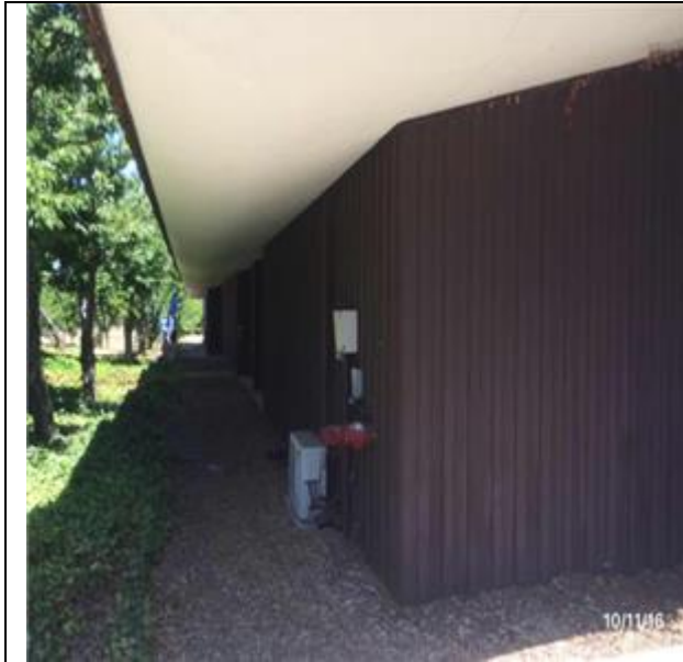
B2011 Exterior Wall Construction:- View of Wood Clapboard Siding
