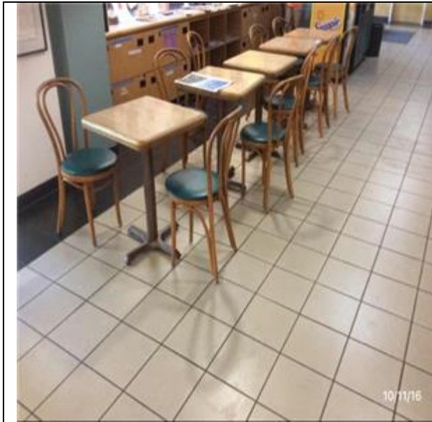
C3024 Flooring:- View of Ceramic Tile
