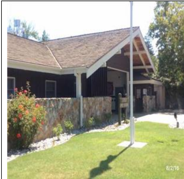
B3016 Gutters and Downspouts:- View of Galvanized Steel Perimeter Gutters & Downspout
