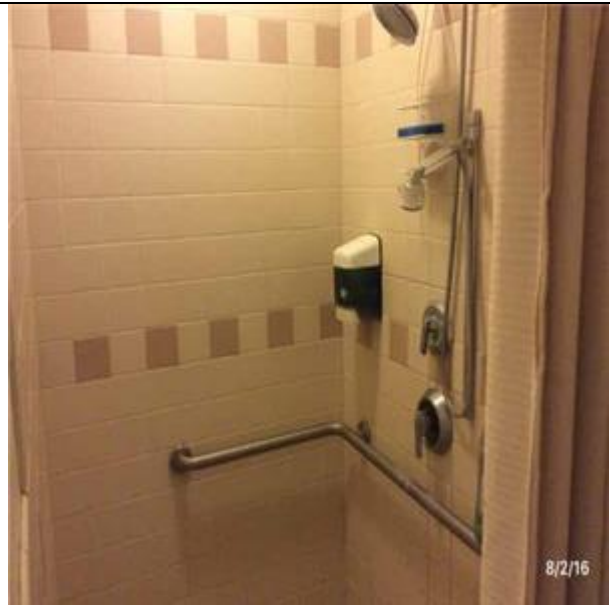
D2017 Showers:- View of Shower - Three Wall Ceramic Tile
