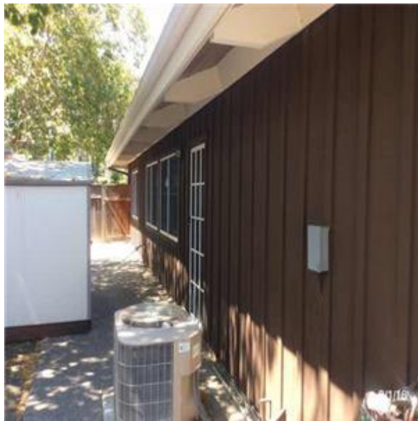
B2011 Exterior Wall Construction:- View of Wood Clapboard Siding
