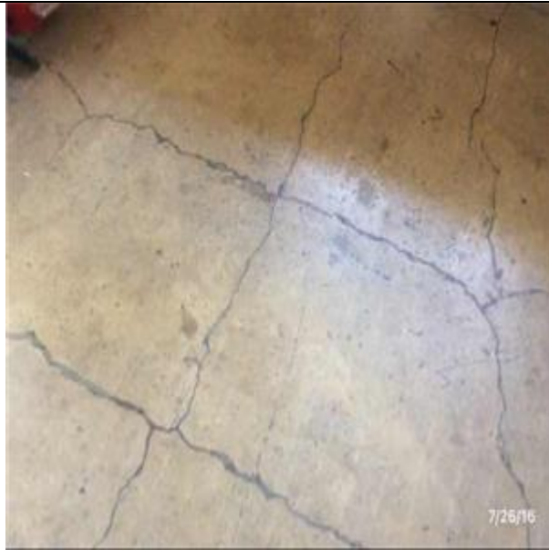
A1031 Standard Slab on Grade:- View of Slab-on-Grade Reinforced Concrete
