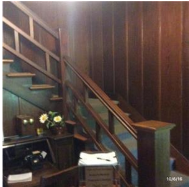
C2011 Regular Stairs:- View of Regular Stairs - Wood Construction to Stage
