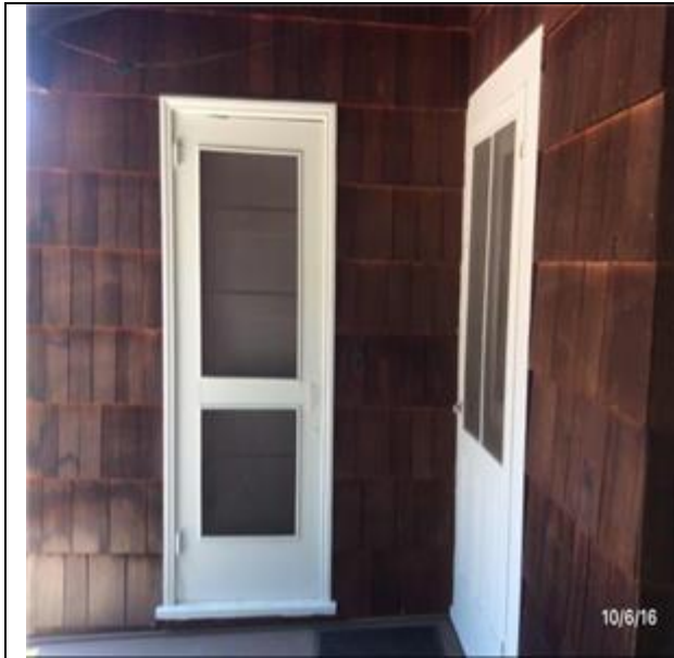
B2039 Other Doors & Entrances:- View of Exterior Single Wood Door
