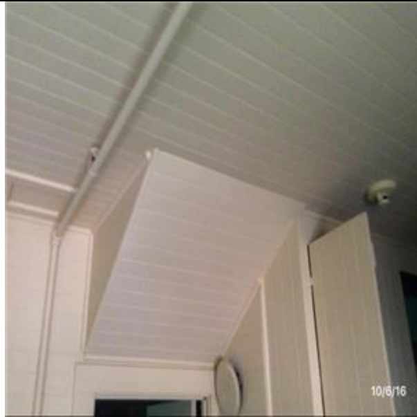
C3031 Ceiling Finishes:- View of Wood Ceiling Painted and Stained
