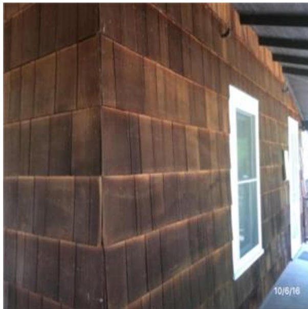
B2011 Exterior Wall Construction:- View of Wood Shingle Siding
