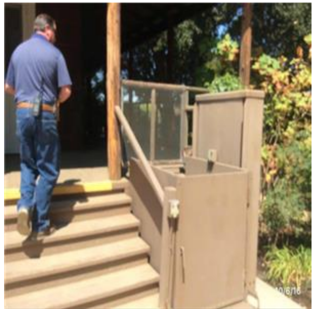
D1094 Conveyors:- View of Wheelchair lift
