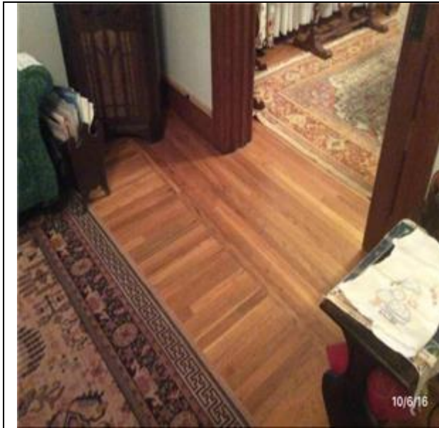
C3024 Flooring:- View of Wood Flooring – Redwood
