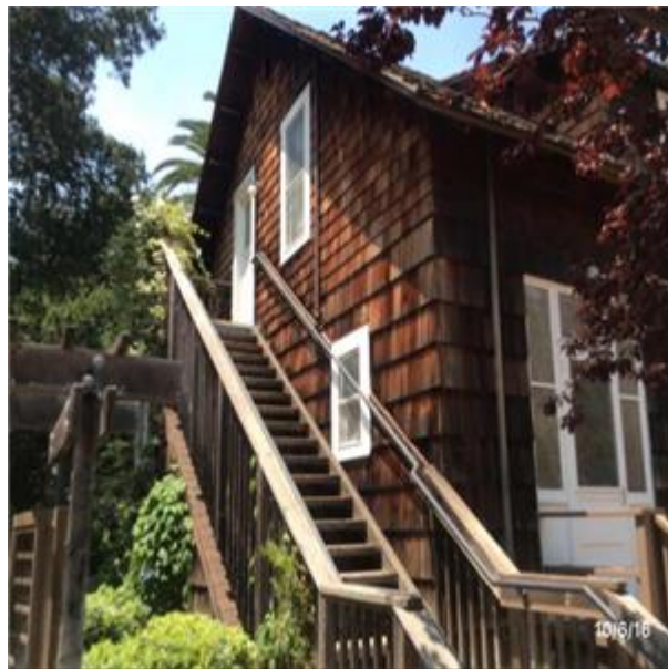
G2033 Exterior Steps:- View of Exterior Wood Steps
