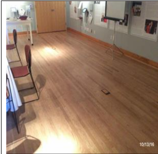
C3024 Flooring:- View of Wood Flooring
