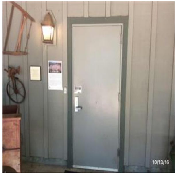
B2039 Other Doors & Entrances:- View of Single HM Doors
