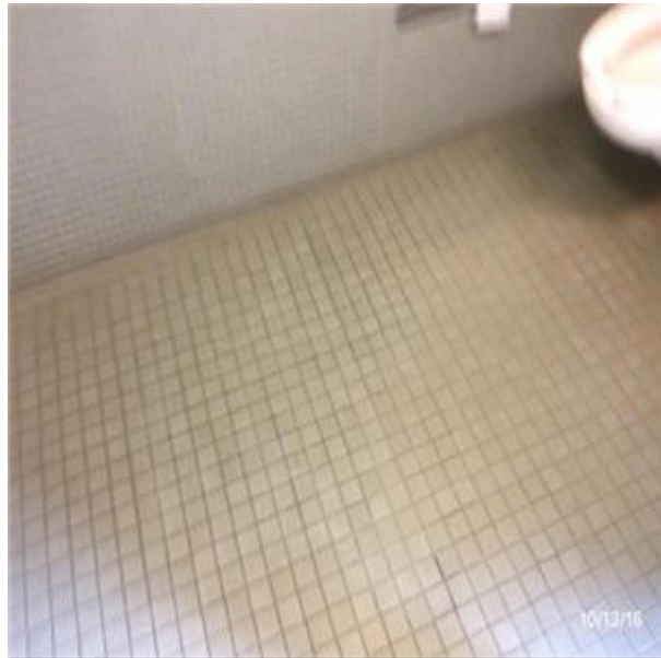
C3024 Flooring:- View of Ceramic Tile
