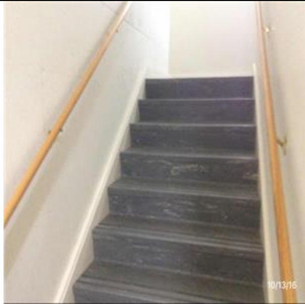
C2011 Regular Stairs:- View of Regular Stairs - Wood Construction
