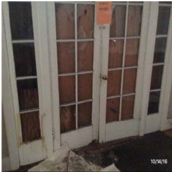
B2039 Other Doors & Entrances:- View of Double Wood Glazed Doors
