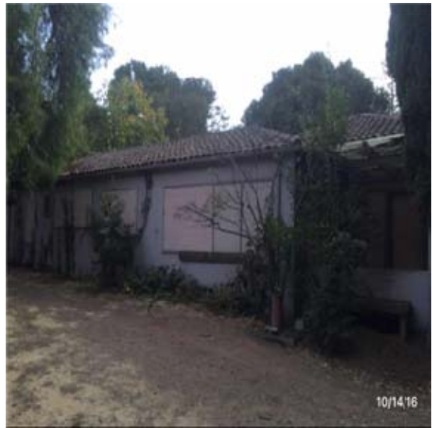
B3011 Roof Finishes:- View of Clay Roof Tile
