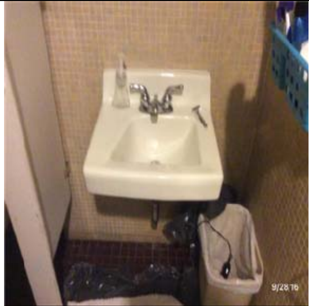
D2013 Lavatories:- View of Wall Hung Lavatories
