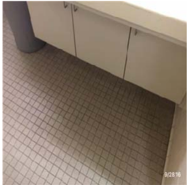
C3024 Flooring:- View of Ceramic Tile
