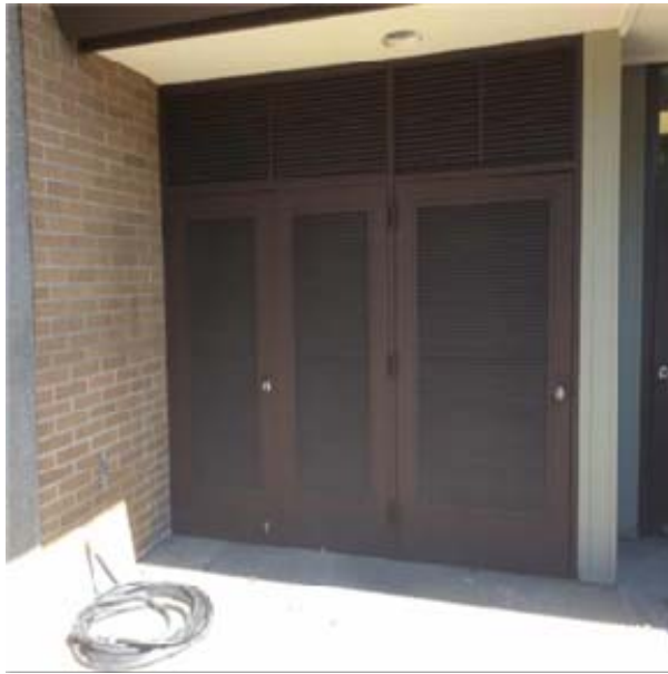
B2039 Other Doors & Entrances:- View of Single HM Louvered Doors
