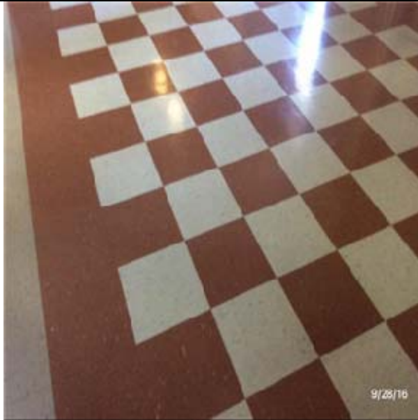
C3024 Flooring:- View of Vinyl Composite Tile (VCT)
