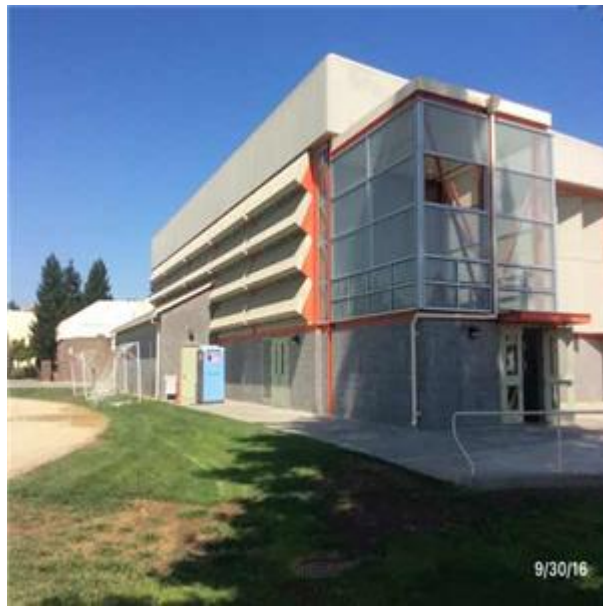
B2011 Exterior Wall Construction:- View of EIFS (Synthetic Stucco) Wall Panels - Standard
