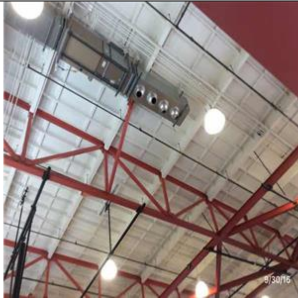
B1021 Flat Roof Construction:- View of Roof Construction - Structural Steel Beams and Joist with Timber Roof Deck
