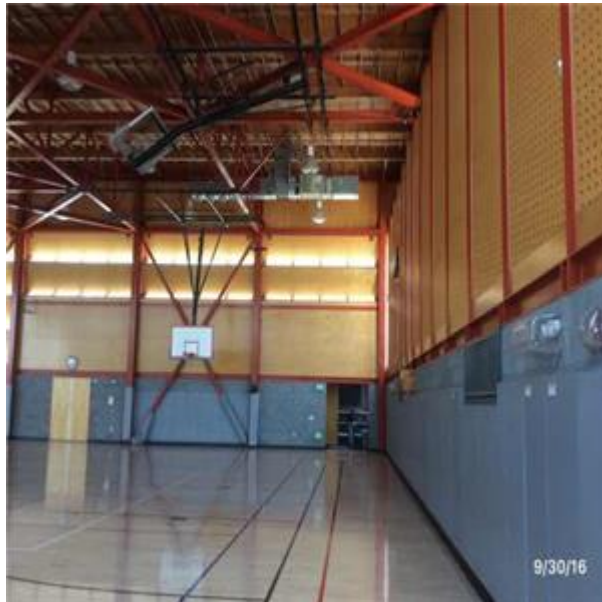
D3021 Boilers:- View of Furnace – Gas
