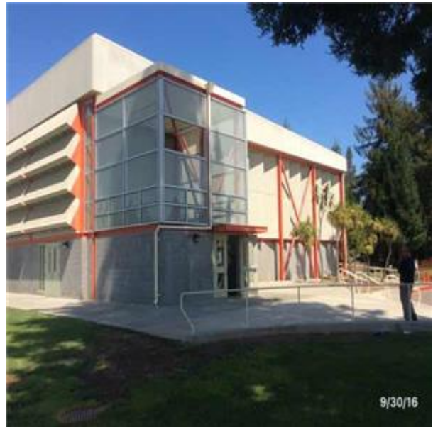
B3016 Gutters and Downspouts:- View of Galvanized Steel Perimeter Gutters & Downspout
