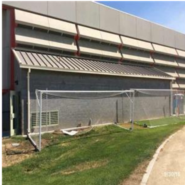
B3011 Roof Finishes:- View of Standing Seam Metal Roof Panels
