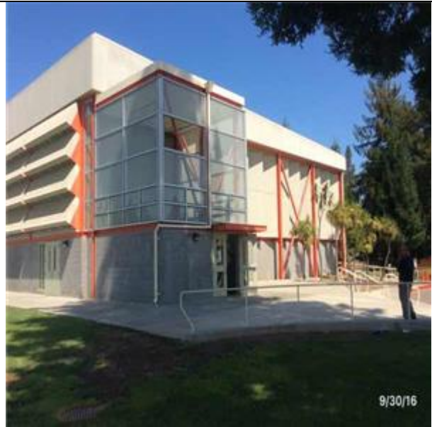
B1031 Steel Frame Structure:- View of Structural Steel Columns and Beams Frame
