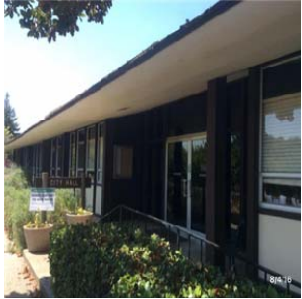
B2016 Exterior Soffits:- View of Exterior Soffits
