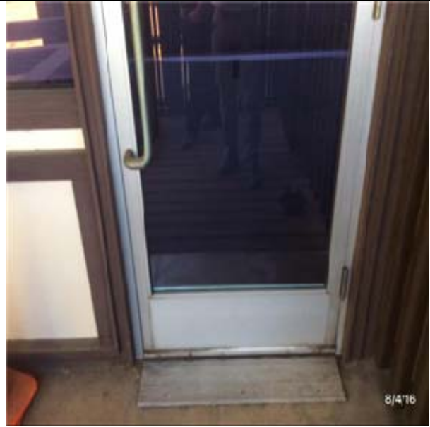
B2031 Glazed Doors & Entrances:- View of Single Aluminum Glazed Doors
