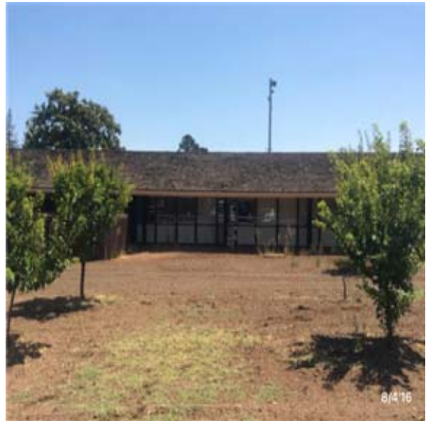
B3011 Roof Finishes:- View of Wood Shake Roof
