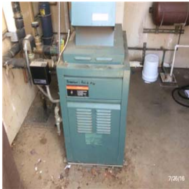
D3032 Direct Expansion Systems:- View of Split-System (Indoor Furnace Unit) 251 to 350 BTU
