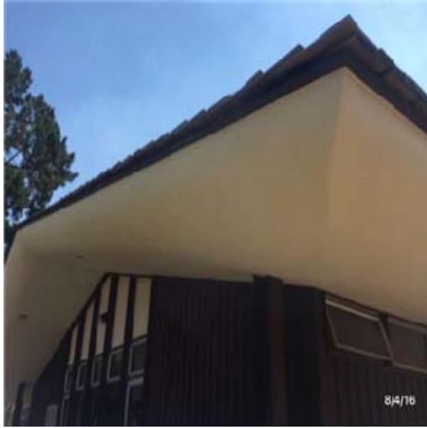
B2016 Exterior Soffits:- View of Exterior Soffits
