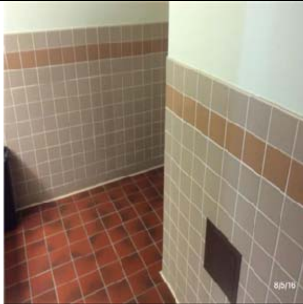
C3012 Wall Finishes to Interior Walls:- View of Ceramic Wall Tiles
