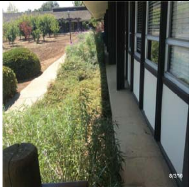
B2011 Exterior Wall Construction:- View of Insulated wall panels to glazing
