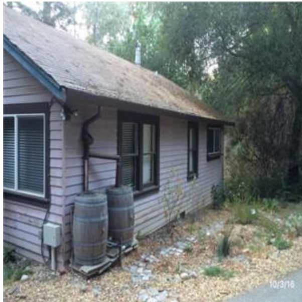
B3011 Roof Finishes:- View of Asphalt Shingle Roof
