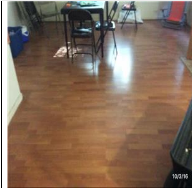
C3024 Flooring:- View of Laminate Wood Floors
