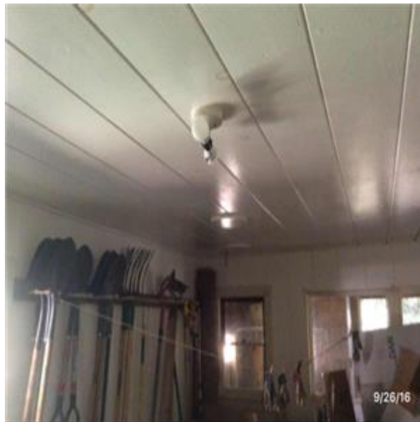
C3031 Ceiling Finishes:- View of Wood Ceiling Painted
