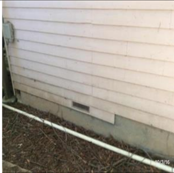
A1011 Wall Foundations:- View of Reinforced Concrete Strip Footing
