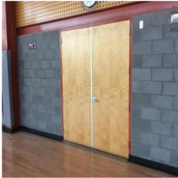
C1021 Interior Doors:- View of Interior Double Wood Door(s)
