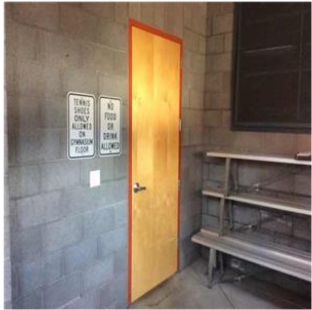
C1021 Interior Doors:- View of Interior Single Door Door(s)
