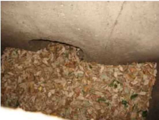
Drain from the previous picture - full of leaves
