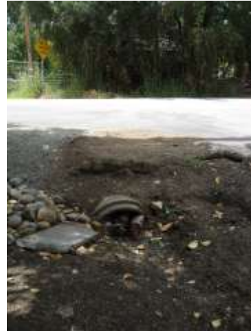
Facing northwest, drain blocked
