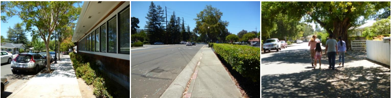
Concrete sidewalk with tree pits in Loyola Corners (left), concrete sidewalk with vertical curb on Fremont Road (center), and gravel/dirt sidewalk on Carob Lane (right).
