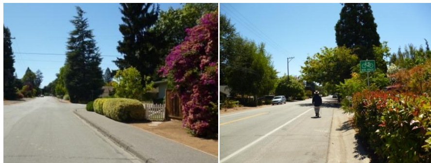
Asphalt berm separating pedestrian walkway (left) and rolled curb with no sidewalk (right).
