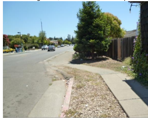
Sidewalks are inconsistent throughout much of Los Altos. Above, a paved sidewalk drops off into a paved shoulder on Miramonte Avenue at Loraine Avenue in the Loyola Corners neighborhood.
