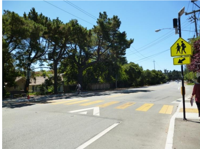
A crossing on Grant Road at Morton Avenue includes curb ramps, a raised crosswalk, yellow ladder striping, and pedestrian-activated in-pavement flashing lights. St. Simon Elementary School is located on the west side of the crosswalk. A bus stop for VTA Route 51 is located on the east.
