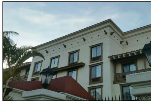
Figure 2: This completely concealed wireless telecommunications facility, including antennas, is cited in the City of San Diego's Land Development Manual in its guidelines for wireless communications facilities.
