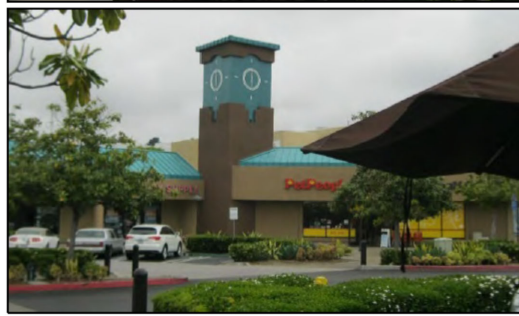
Figure 4: A cupola (above) and a clock tower (below) conceal antennas.
