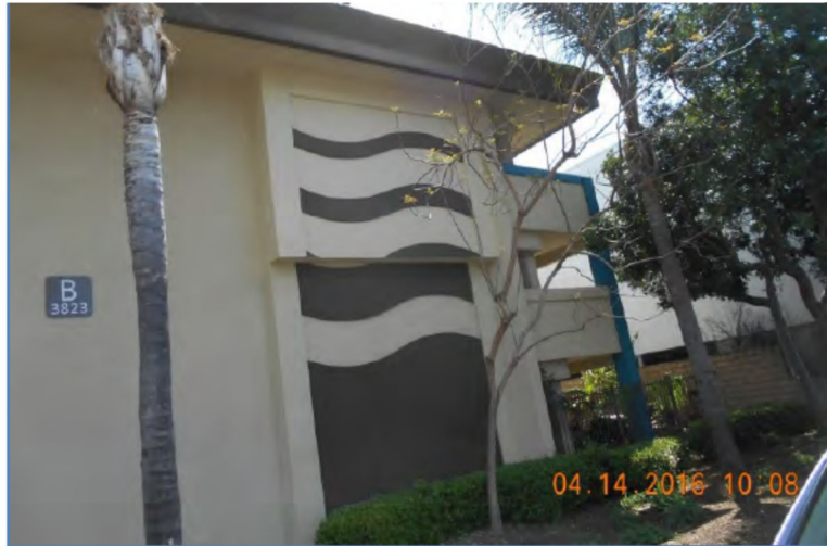
Figure 5: Although façade-mounted boxes are not preferred, this example from San Diego achieves integration with the structure.
