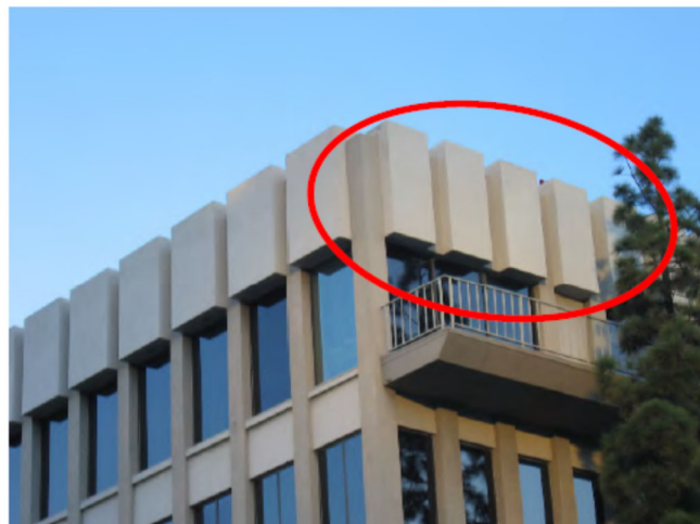
Figure 1: This well-concealed wireless telecommunications facility has its antennas architecturally integrated into the building.
