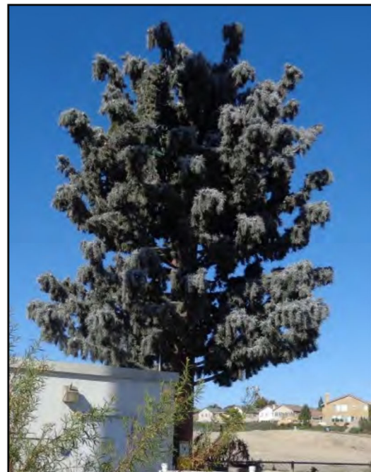
Figure 6: In this example, antennas are concealed by the faux "mono-pine."
