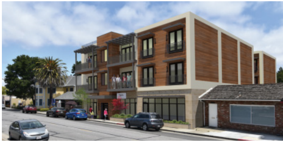
385, 387 & 389 1ST STREET (IN CONSTRUCTION) 4
