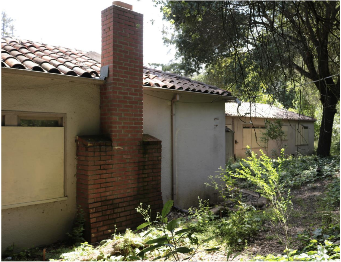
Looking south along the west elevation.
