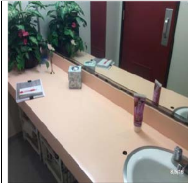
D2013 Lavatories:- View of Vanity Top Lavatories
