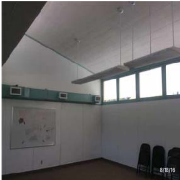
C3012 Wall Finishes to Interior Walls:- View of Wainscot
