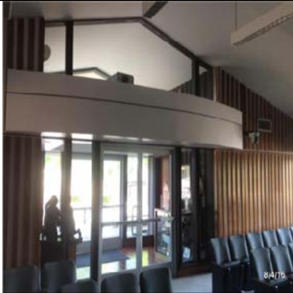
C1011 Fixed Partitions:- View of Plate Glass Wall
