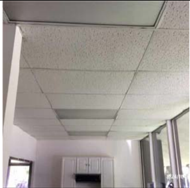
C3032 Suspended Ceilings:- View of Acoustical Tile
