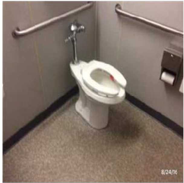
C3024 Flooring:- View of Vinyl Sheet
