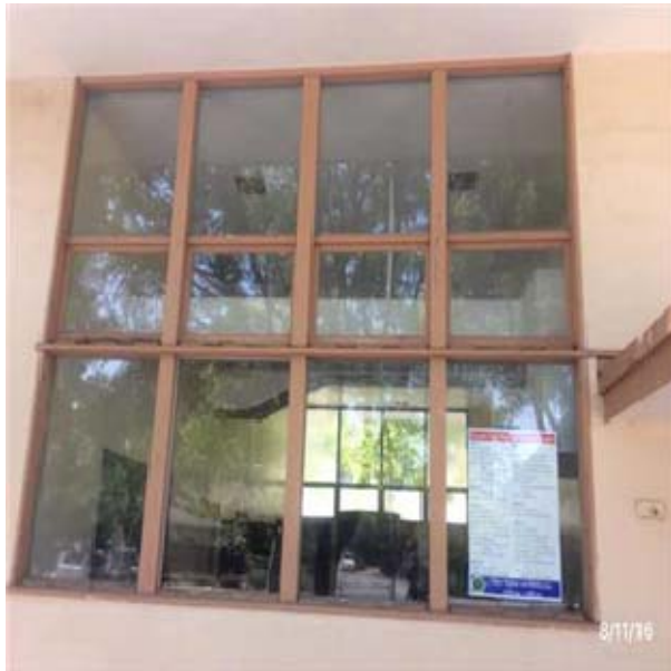
B2021 Windows:- View of Wood Window Units - Fixed or Single Hung
