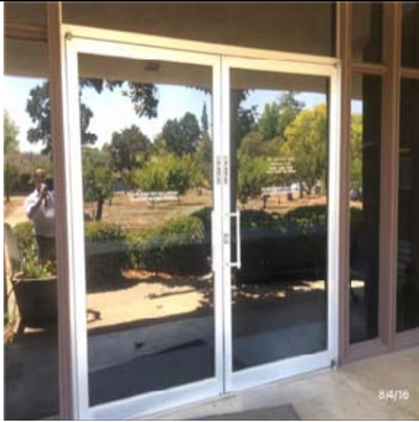
B2031 Glazed Doors & Entrances:- View of Double Aluminum Glazed Doors
