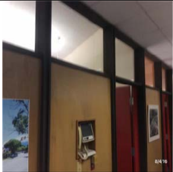
C1011 Fixed Partitions:- View of Wood Veneer and Plate Glass Wall
