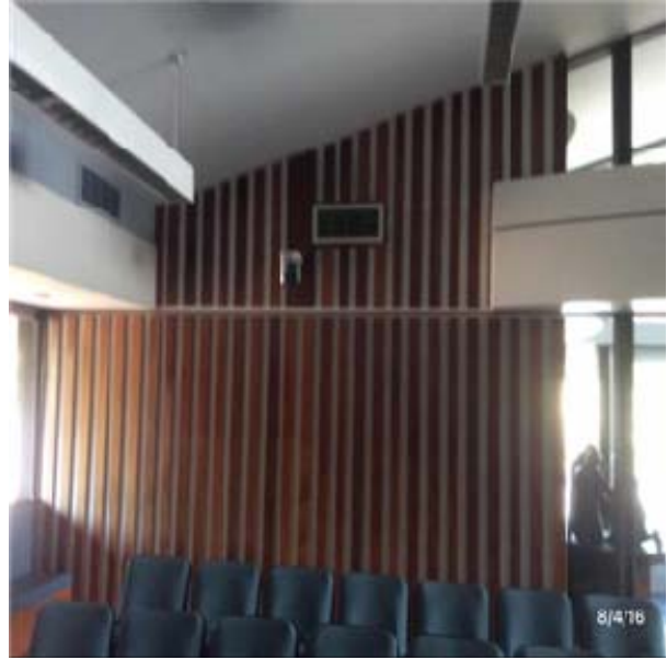
C3012 Wall Finishes to Interior Walls:- View of Wood Panels
