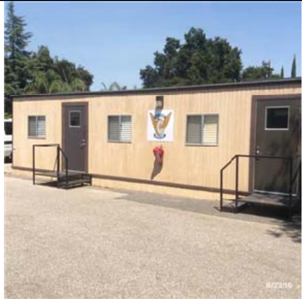
F1012 Pre-engineered Structures:- View of PreFab Modular Building #1
