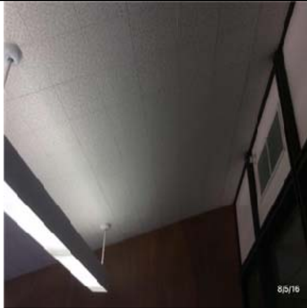
C3032 Suspended Ceilings:- View of Acoustic Ceiling System with Concealed Grid
