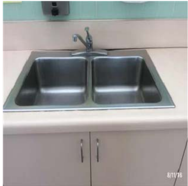
D2014 Sinks:- View of Countertop Double Bowl Kitchen Sinks
