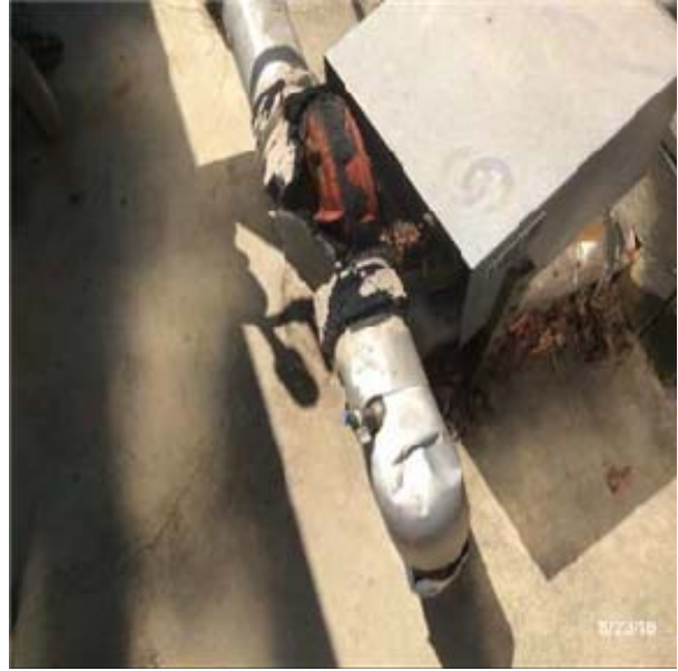
D3045 Chilled Water Distribution:- View of CW Circulation Pump/Motor 1-2 HP
