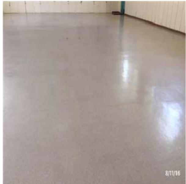
C3024 Flooring:- View of Vinyl Sheet
