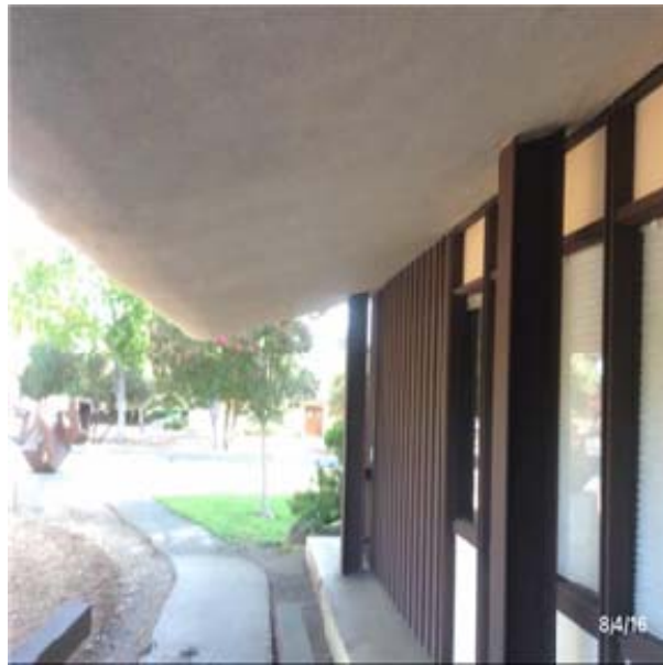
B2011 Exterior Wall Construction:- View of Wood Cladding
