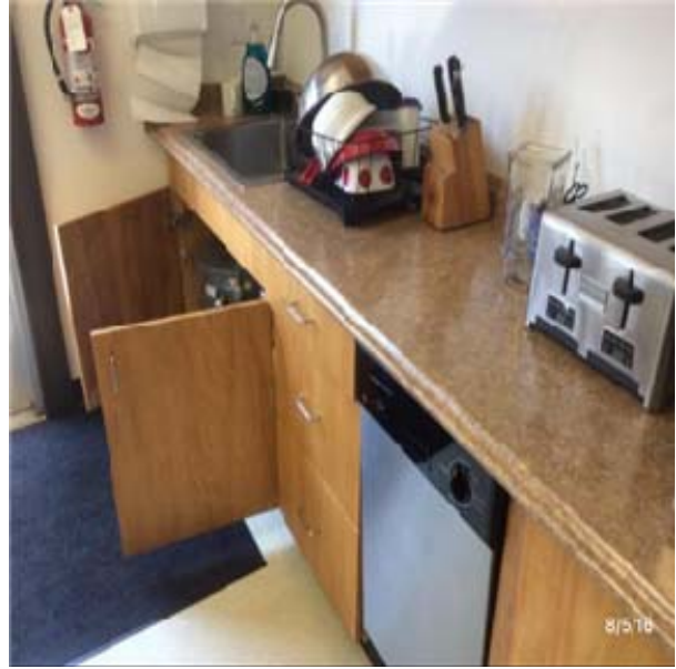
E1095 Unit Kitchens:- View of Unit Kitchens - Counter Top - Laminated
