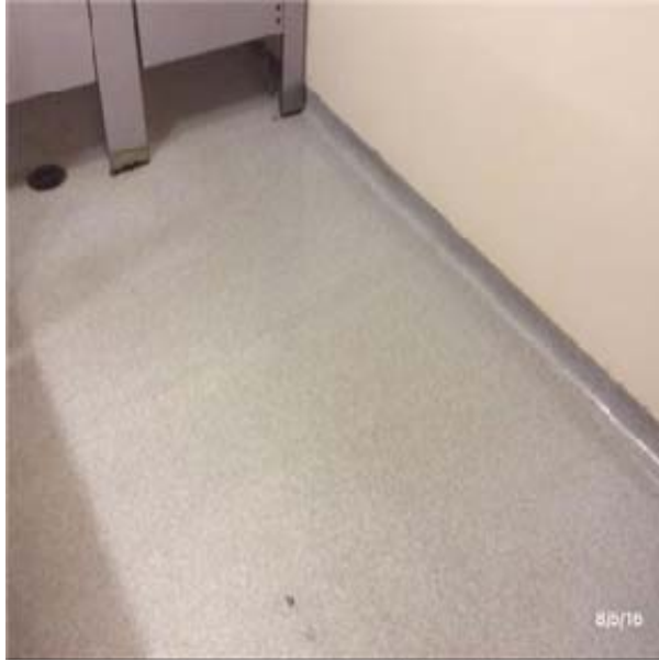
C3024 Flooring:- View of Vinyl Sheet
