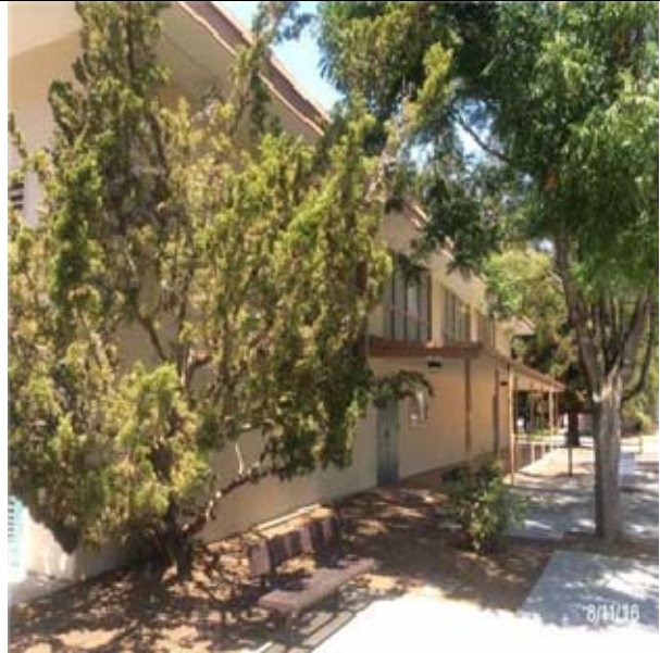
B2011 Exterior Wall Construction:- View of Stucco over Stud Walls
