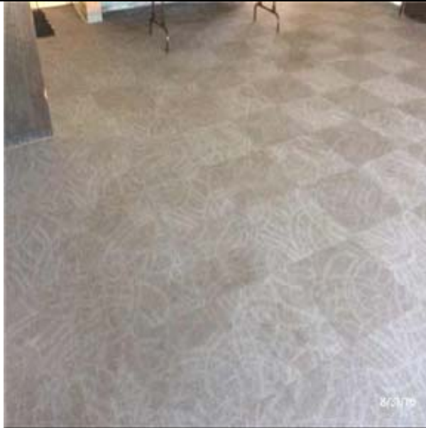
C3025 Carpeting:- View of Carpet Tiles – Standard
