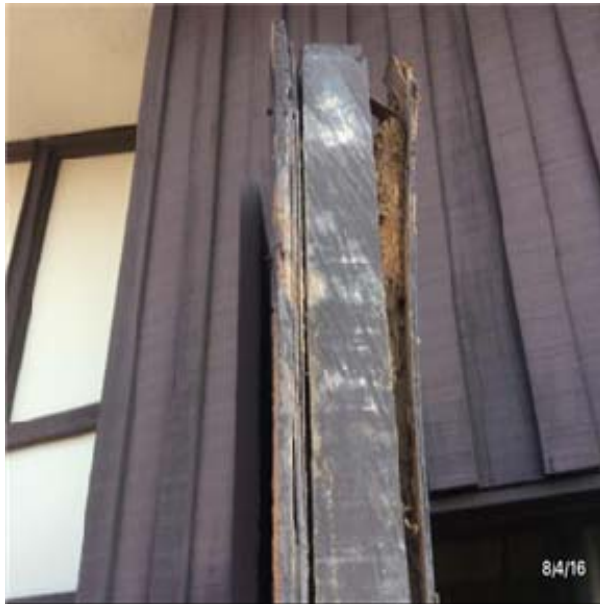
B2039 Other Doors & Entrances:- View of Exterior Double Wood Door(s)
