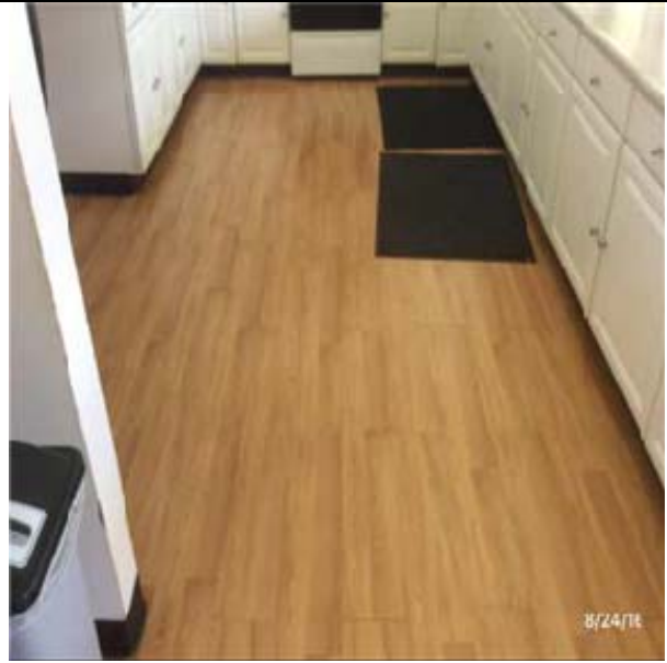
C3024 Flooring:- View of Laminate Wood Floors
