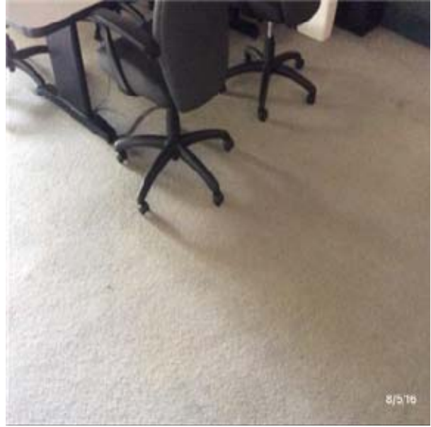
C3025 Carpeting:- View of Carpet Tiles – Standard
