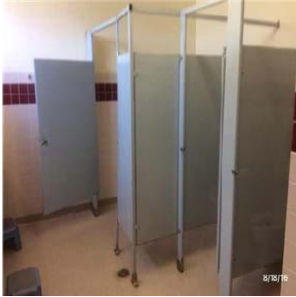
C1014 Site Built Toilet Partitions:- View of Toilet Partition
