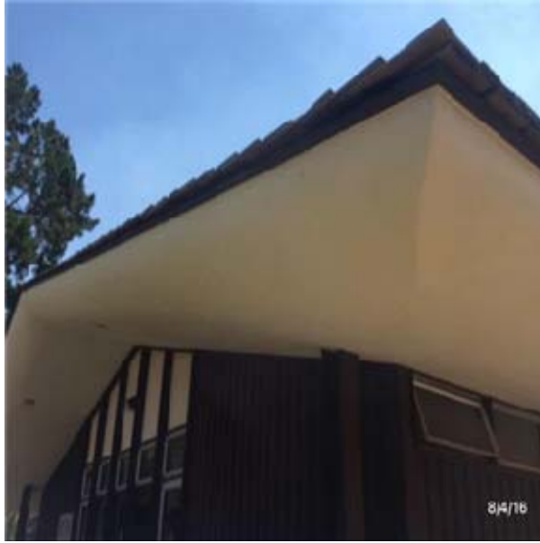
B2016 Exterior Soffits:- View of Exterior Soffits
