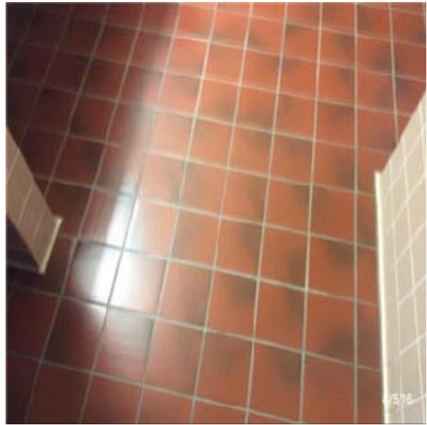
C3024 Flooring:- View of Quarry Tile
