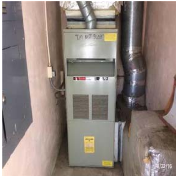
D3032 Direct Expansion Systems:- View of Split-System (Indoor Furnace Unit) 101 to 150 BTU
