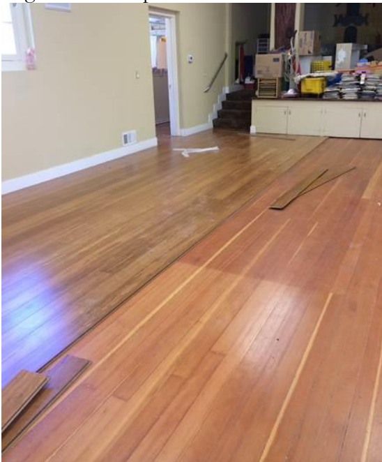
Installation in progress, the new floor is on the left, the original floor on the right.
