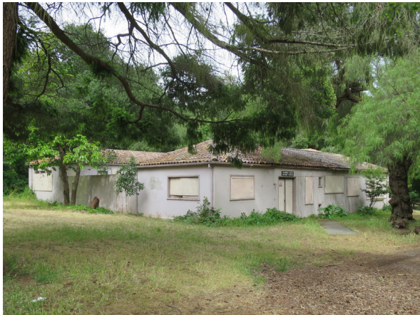
Figure 7. Southeast (left) and northeast (right) elevations, looking west (photo: ARG, May 2019).
