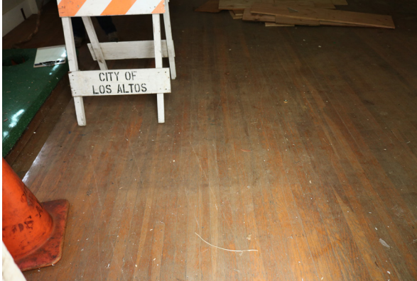
Original wood flooring in the Entry (ARG, 2019).
