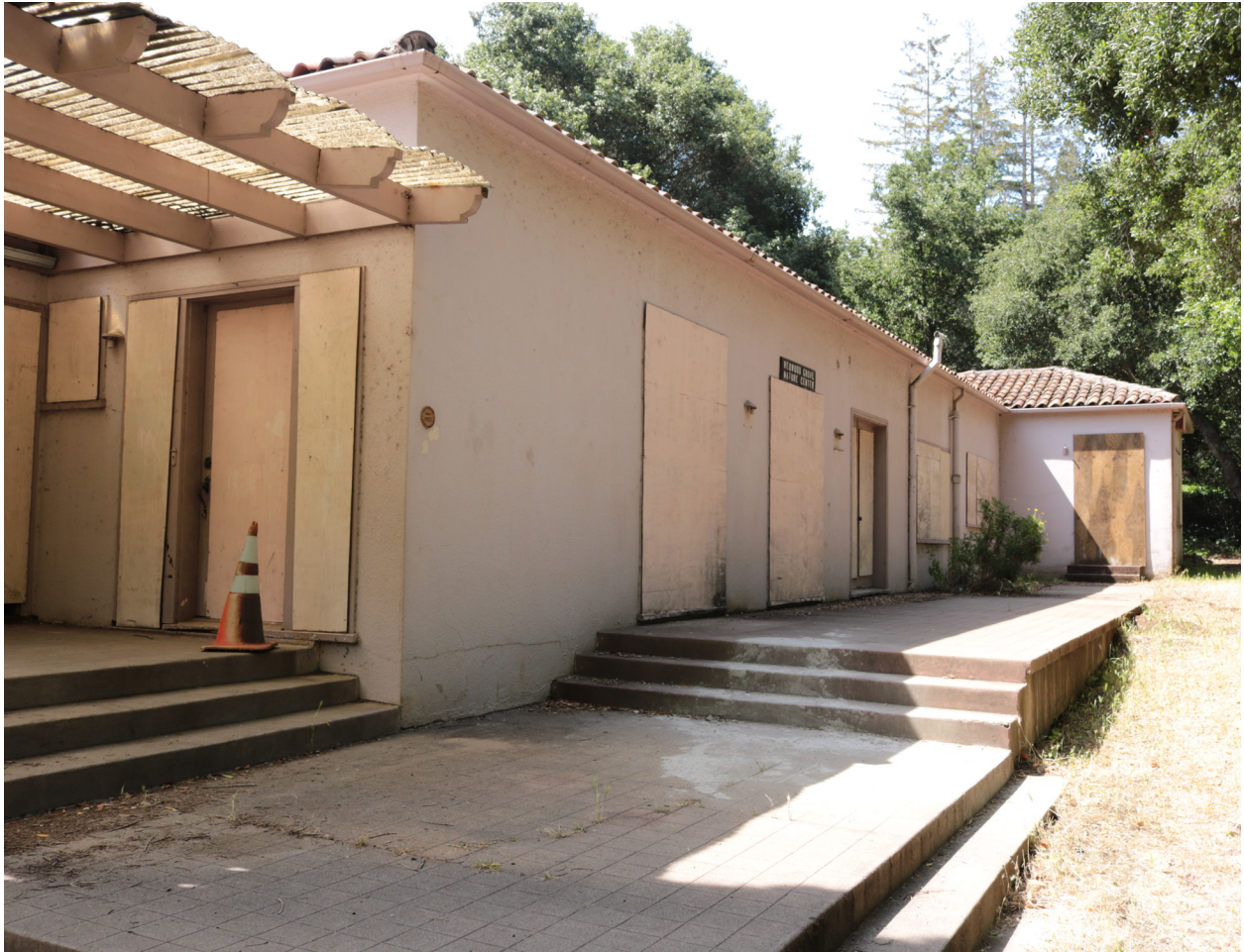
North elevation and patio adjacent to north wall.
