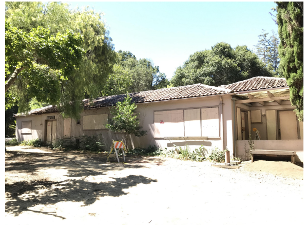
Photo #10 - East Elevation of the East Wing of the Building
