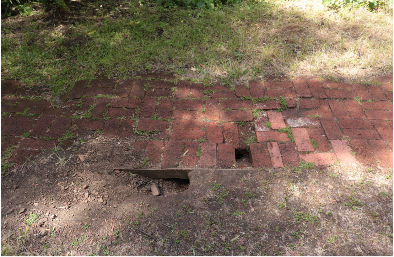
View of walkway paving along east elevation.
