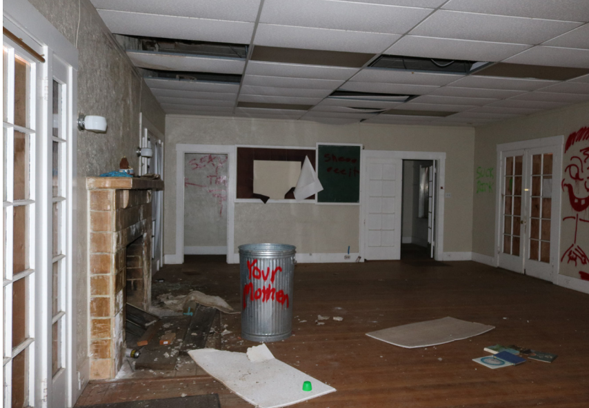
Overall view looking west inside main room.
