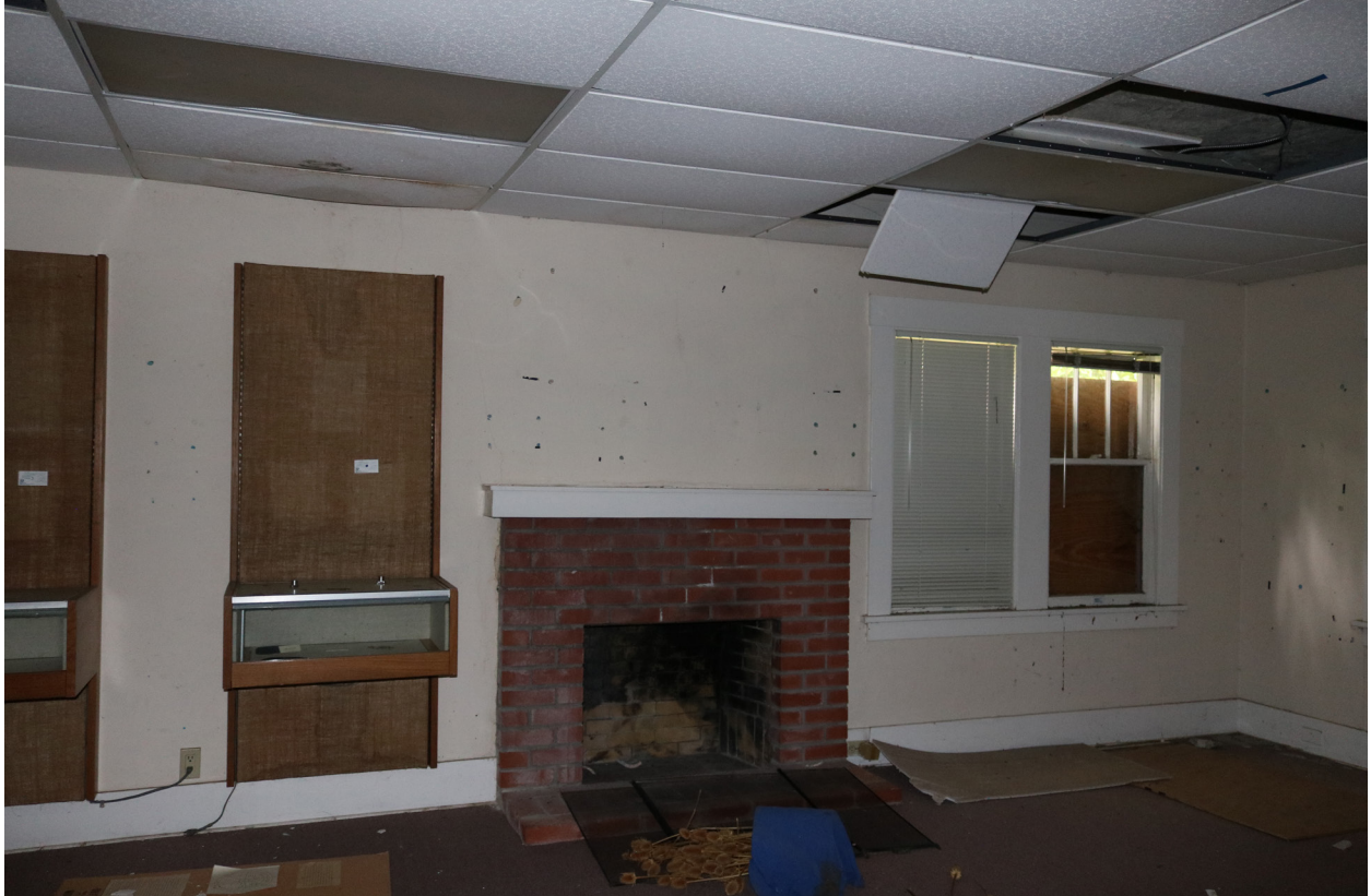
Overall view inside Ohlone room.
