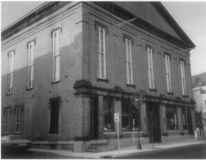
Figure 5. At the Hudson Opera House, a multi-arts center in Hudson, New York, the historic structure report was prepared incrementally. The first phase of the report focused on assessment and recommendations for repair of the roofing, the most critical issue in preservation of the building. Photo: Gary Schiro.
