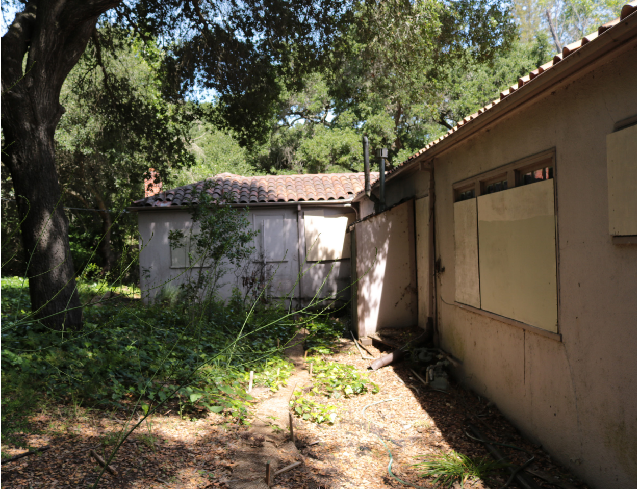
Looking north along the west elevation.
