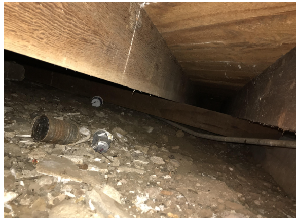
Photo #16: Isolated Concrete Footing at North and South Sections of Lodge
