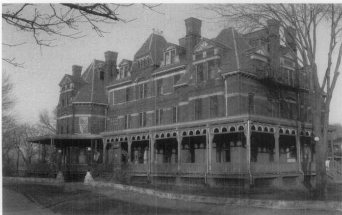
Figure 15. The historic structure report for the Hotel Florence, shown here in 1886 (upper), 1963 (center), and 2004 (lower) views, provided a basis for stabilization and repair work which has been completed. Initial phases of work addressed preservation of the building envelope, structural repairs, and limited mechanical and electrical improvements. The report also provided recommendations for future rehabilitation work that will be implemented in phases as funding becomes available. Photos: upper and center, Historic American Building Survey; lower, Wiss, Janney, Elstner Associates, Inc.
