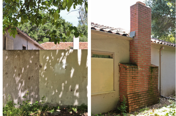
Dissimilar paint colors along the south elevation (left); biological growth at the west chimney (right); (ARG, 2019).
