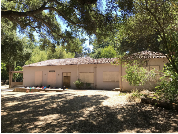
Photo #1 - North Elevation of the Building
