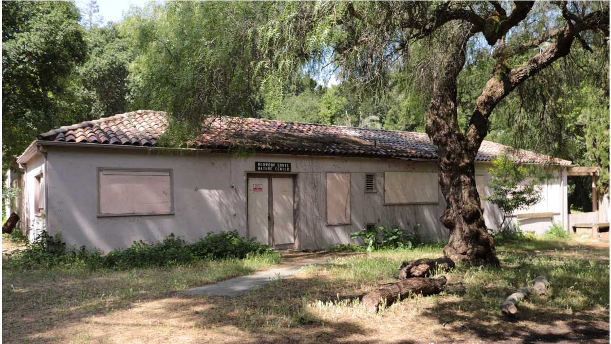
Overall view of east elevation.
