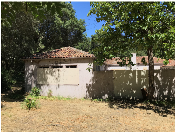
Photo #5 - South Elevation of the West Wing of the Building
