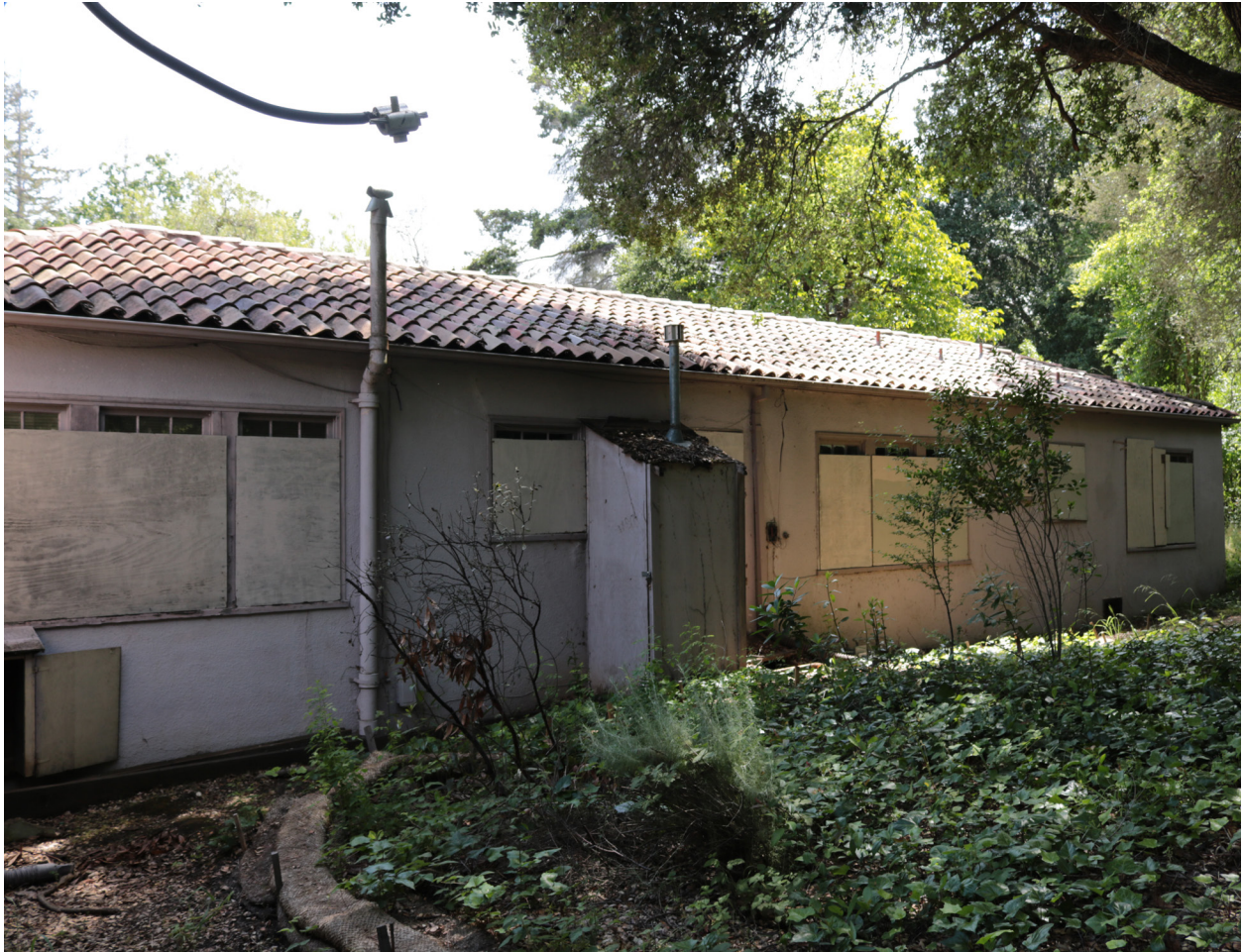
Overall view at center of west elevation, looking southeast.
