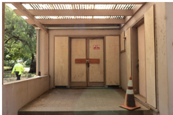
Figure 3. Primary entry porch (photo: ARG, May 2019).
