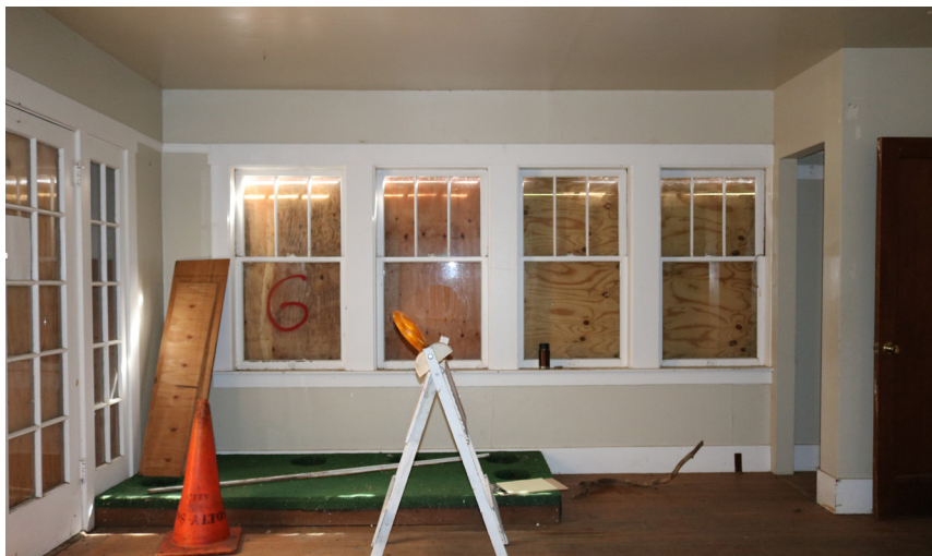
Looking north east inside the entry.
