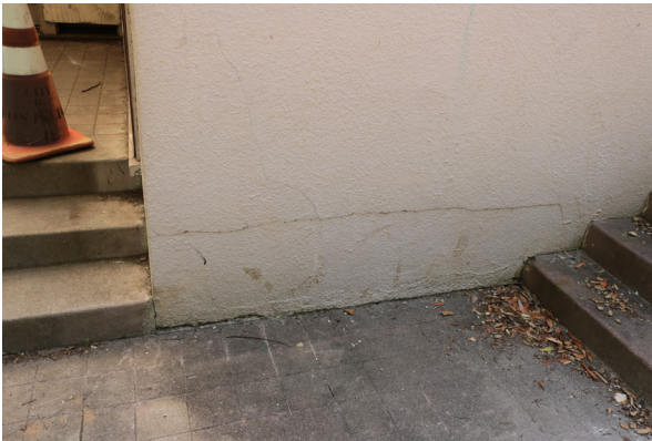
Crack along the base of the north elevation at the Main Entry (ARG, 2019).
