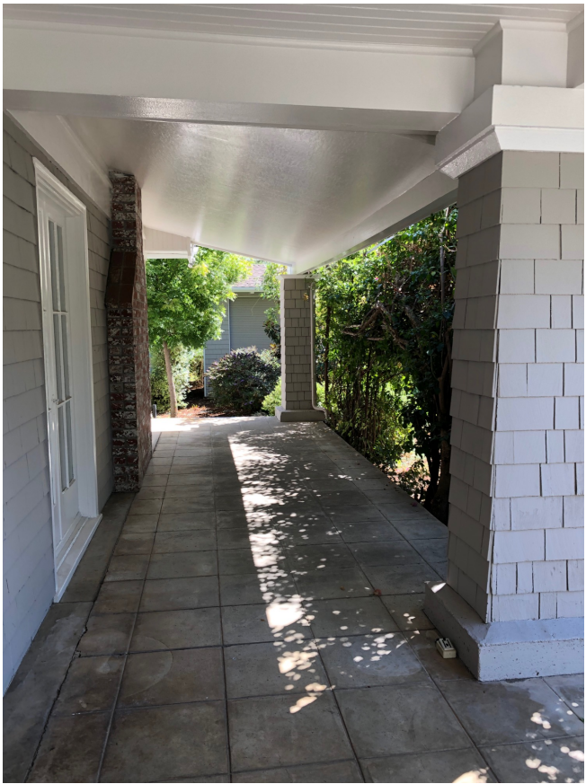
Front Covered Porch
