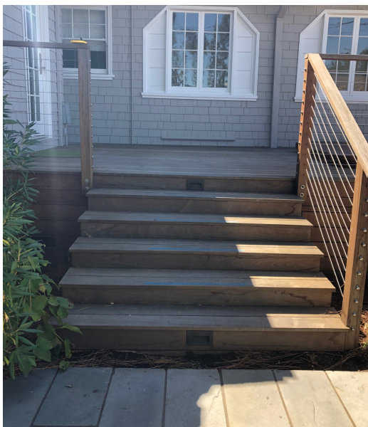
Rear Wood Deck
