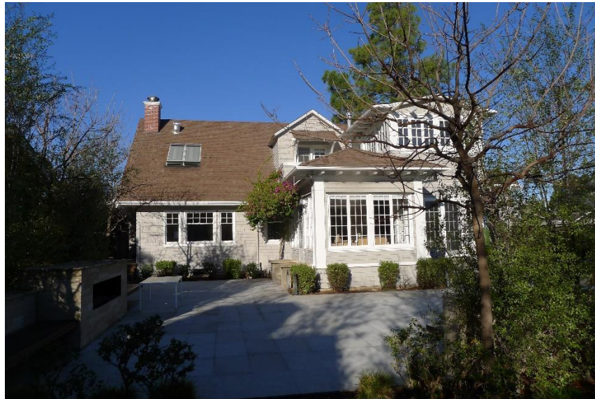
East Elevation Showing New Skylights
