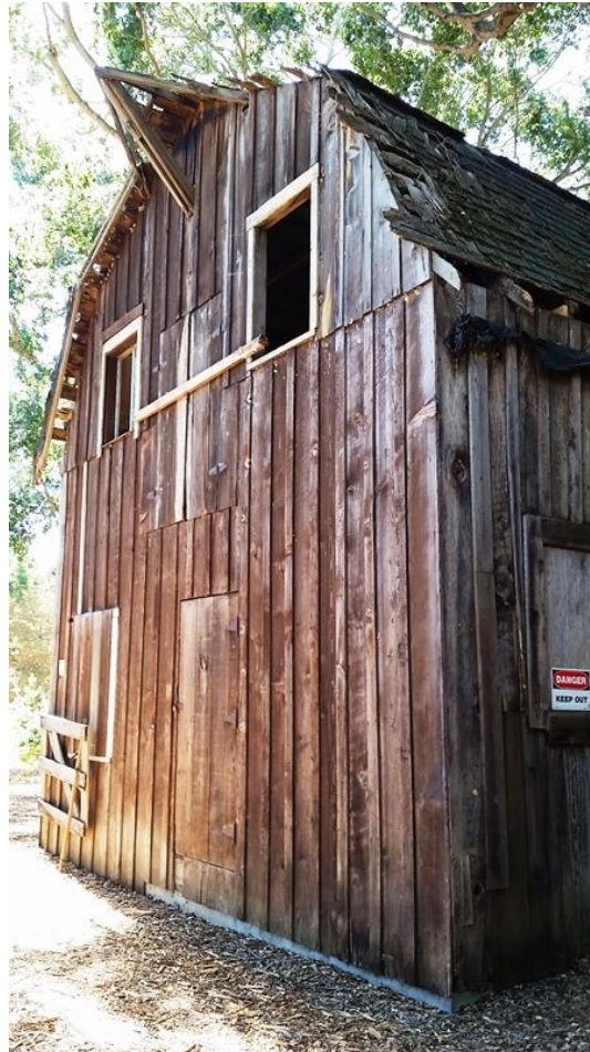
North Elevation, viewed facing southeast.
