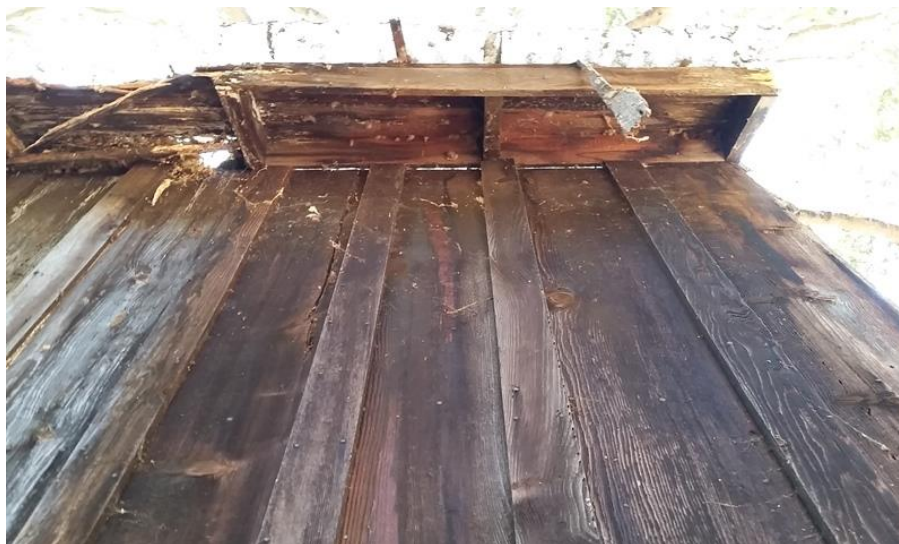
Detail of Eaves - West Elevation, viewed facing east.
