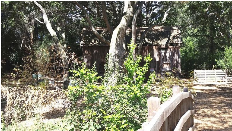
East Side of Barn concealed in its setting, viewed facing west across Adobe Creek.
