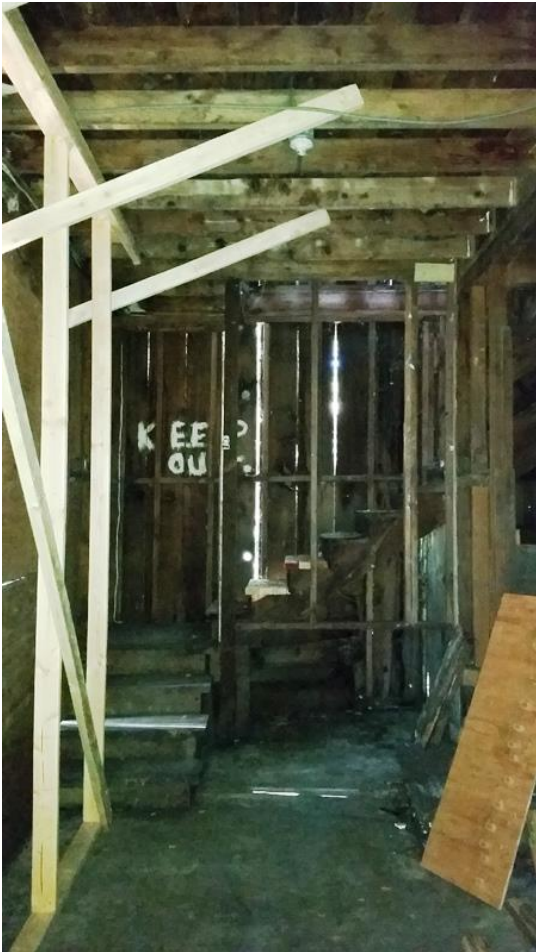
First Floor Interior, viewed facing south.
