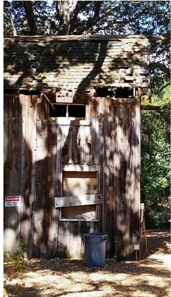
Detail of Northeast Wall, viewed facing west.
