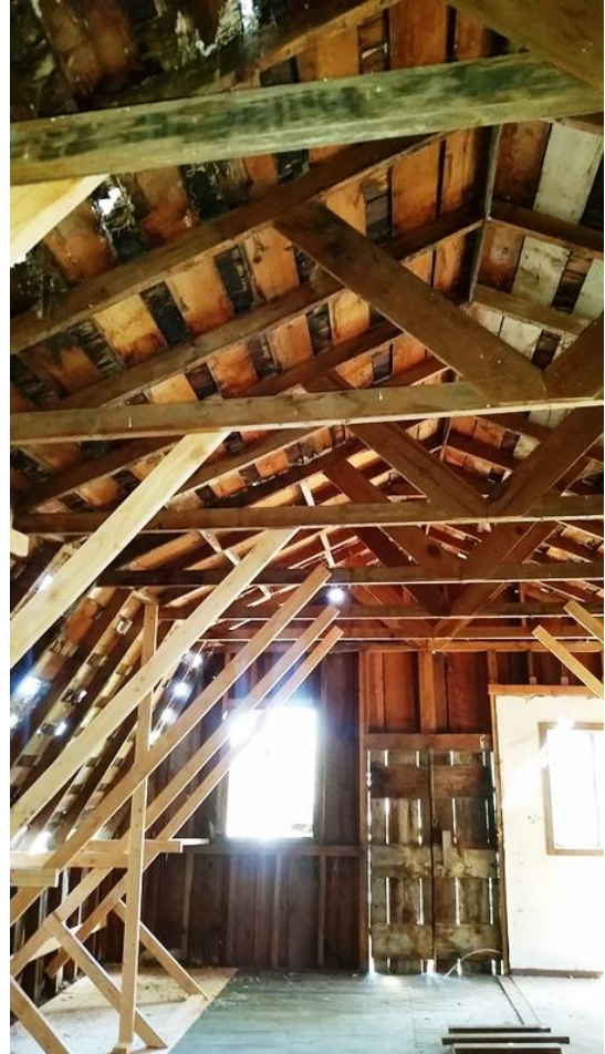
Second Floor Interior, viewed facing north.
