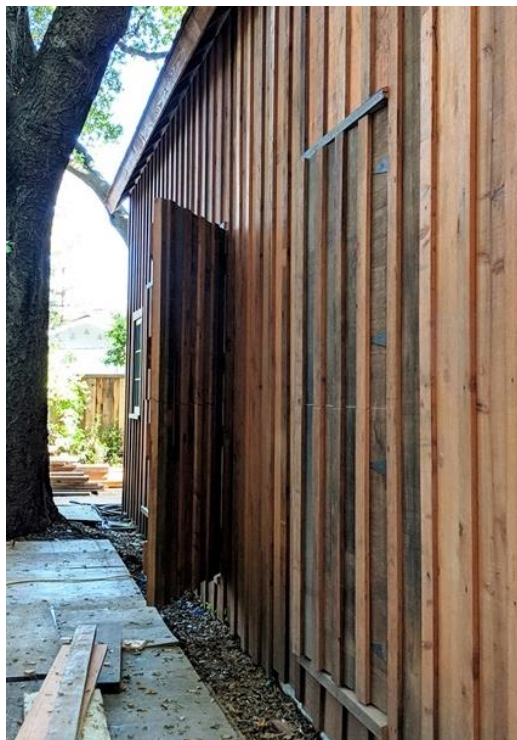
Detail of Rehabilitated Stall Doors. Facing north. Image by Leslie Dill. April 2019.
