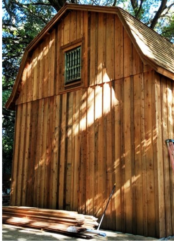
View of South elevation, facing northwest. Image by Leslie Dill. April 2019.
