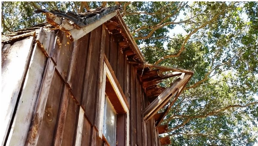
Hay Hood Detail - North Elevation, viewed facing west.
