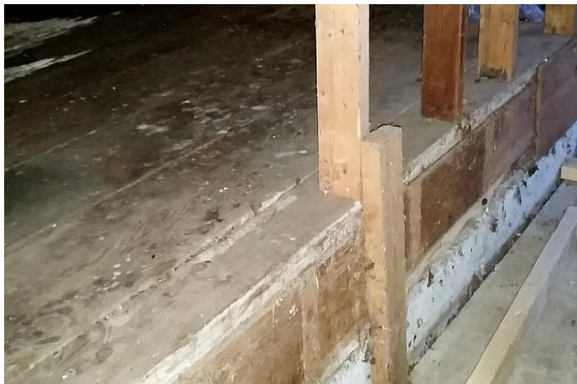
First Floor Raised Floor Framing, viewed facing northwest.
