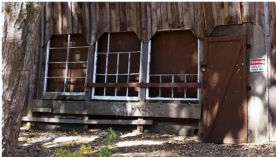
Detail of East Windows, viewed facing west.
