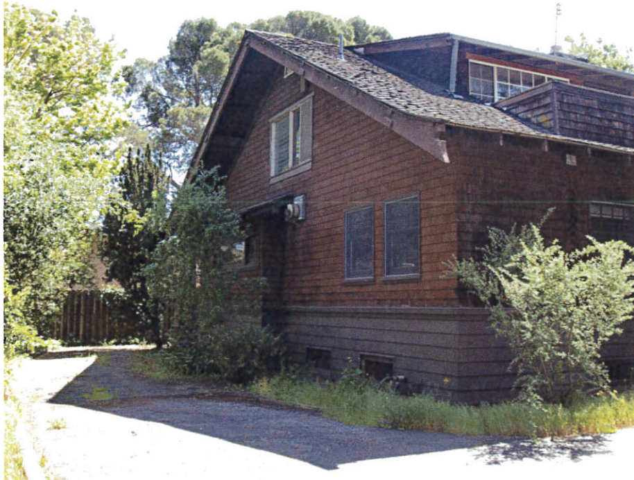
North Elevation, viewed facing southeast.
