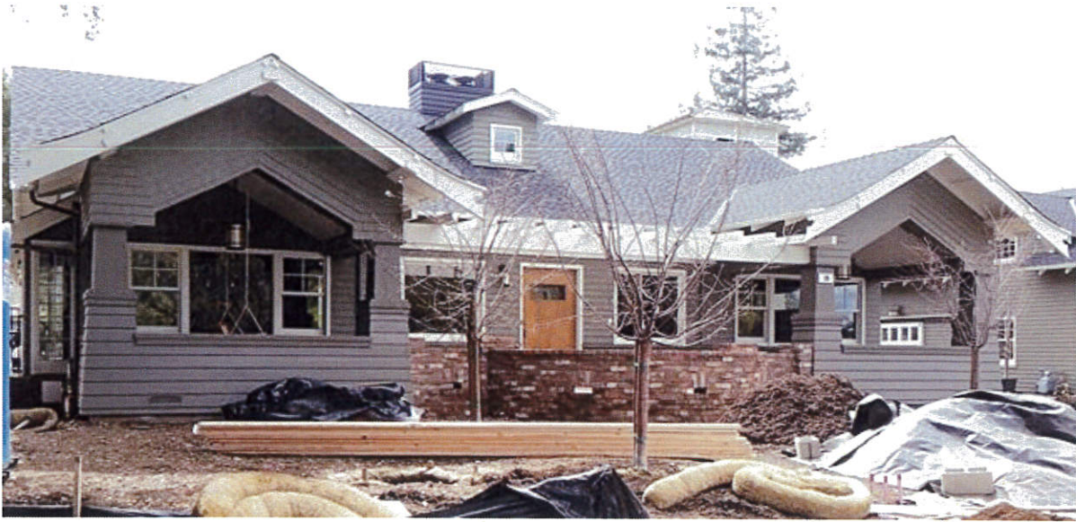
Front Façade, viewed facing southwest
