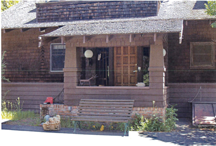
Rear entry (now main entry), viewed facing east.
