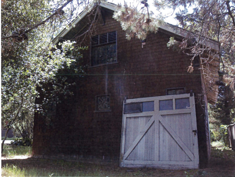
Carriage house/garage, viewed from Yerba Buena Avenue.
