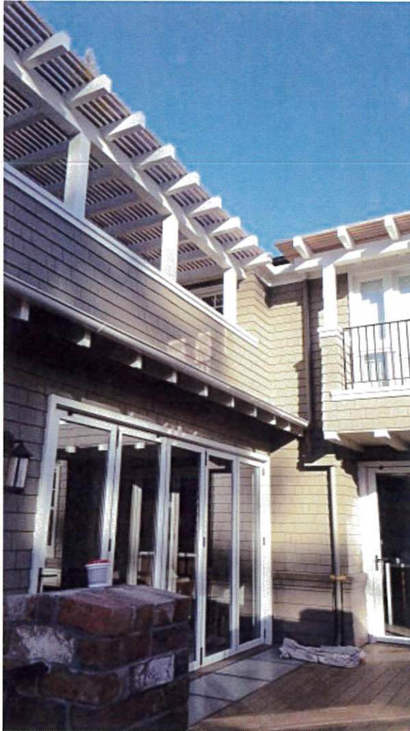
Rear of House, from the southwest, showing rehabilitated dormer and new rear door
