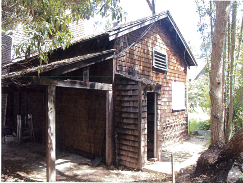
Rear view of addition to tank house, viewed facing northeast.
