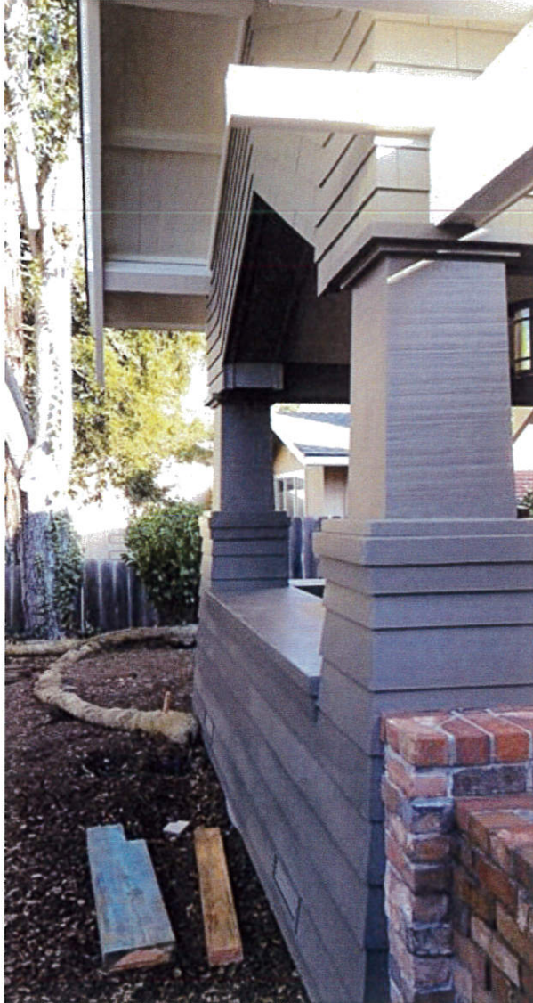
Detail of east gable wall
