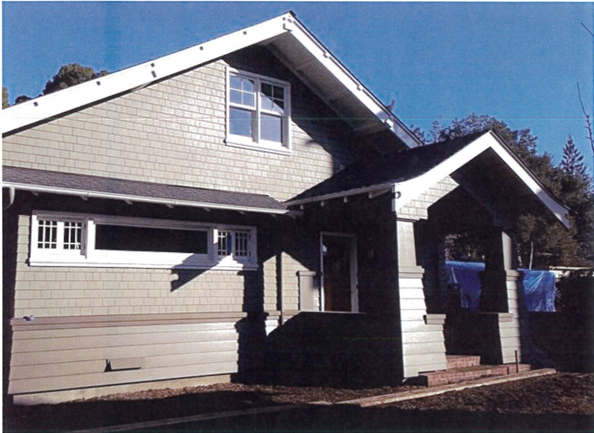
West Side, viewed facing southeast
