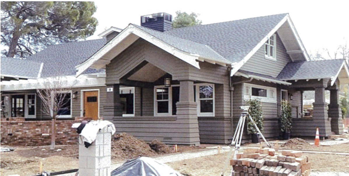
Front Façade, viewed facing southeast
