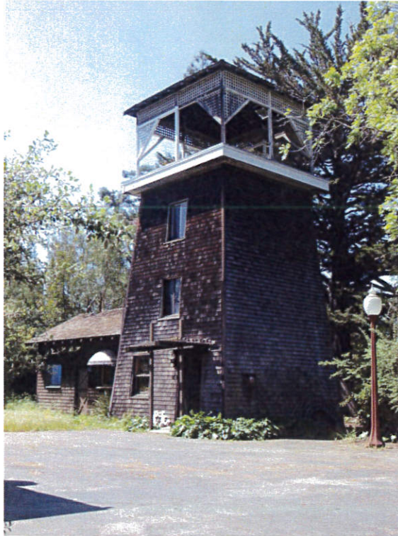
Tank house, viewed facing southwest.
