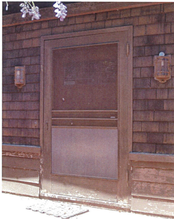
Original front entry door, viewed facing southwest.
