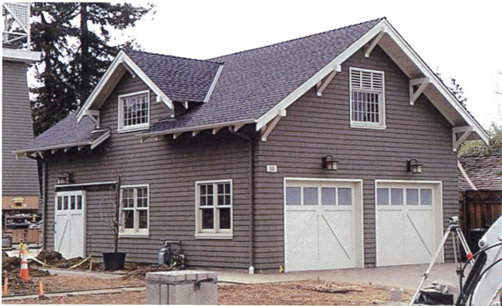
Carriage House/Garage, from the northeast
