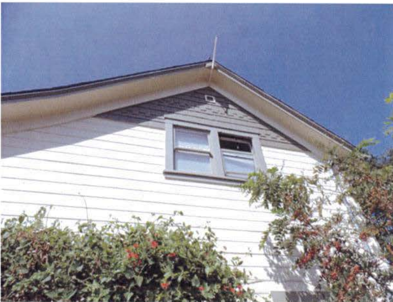
Figure 3. Detail of decorative wood shingles at eastern elevation (Garavaglia Architecture, Inc., August 2015)
