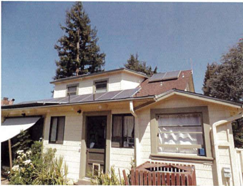
Figure 13. South elevation at rear of home with gabled addition to the right and enclosed kitchen to the left. Door and center windows comprised the original kitchen (Garavaglia Architecture, Inc., August 2015)
