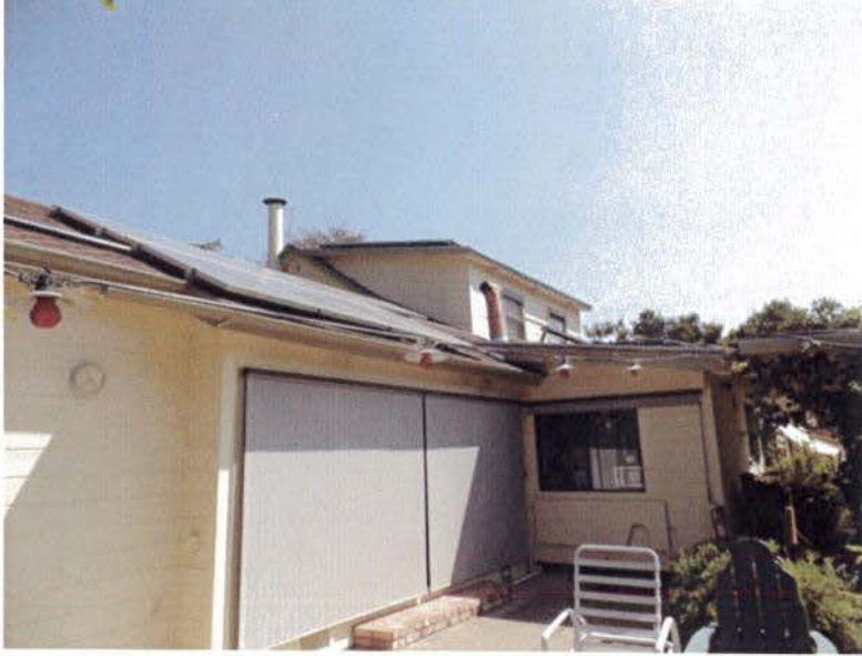
Figure 6. South elevation with Pool Room addition to the left and enclosed porch/kitchen addition to the right with overhang (Garavaglia Architecture, Inc., August 2015)
