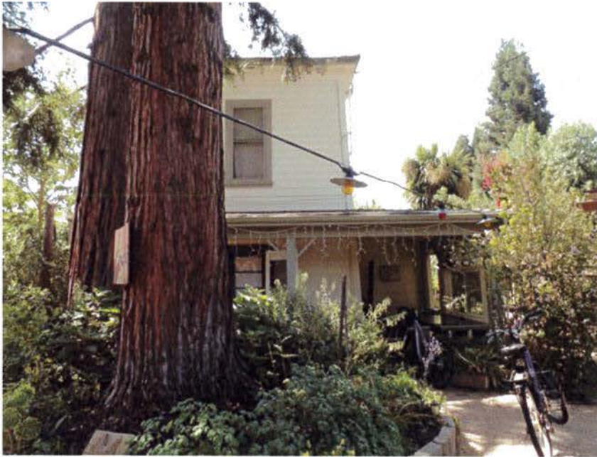
Figure 22. North elevation of the Water Tower with partial wraparound porch and first story addition to the right. Note two mature Redwood trees to the left. (Garavaglia Architecture, Inc., August 2015)
