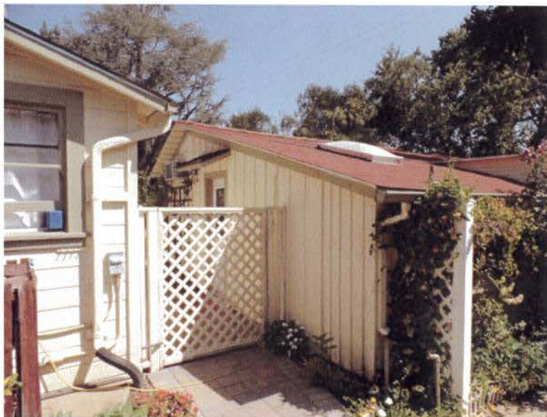
Figure 13. West elevation of Garage addition with skylight. Note lattice fence between the main house and the Garage (Garavaglia Architecture, Inc., August 2015)
