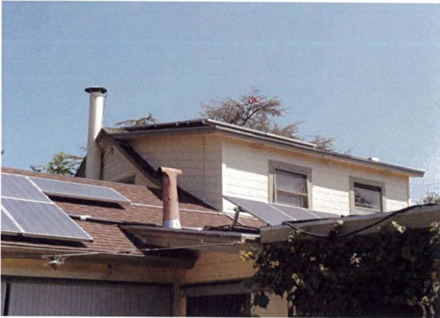
Figure 15. Northeast view of roofline. Note the original second story portion of the home with the Pool House addition to the left and the enclosed porch/kitchen addition to the right (Garavaglia Architecture, Inc., August 2015)
