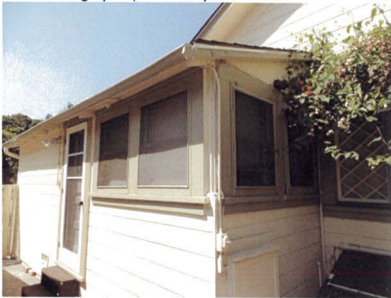
Figure 4. Detail of side addition at eastern elevation. Note the difference in siding material and window at right (Garavaglia Architecture, Inc., August 2015)
