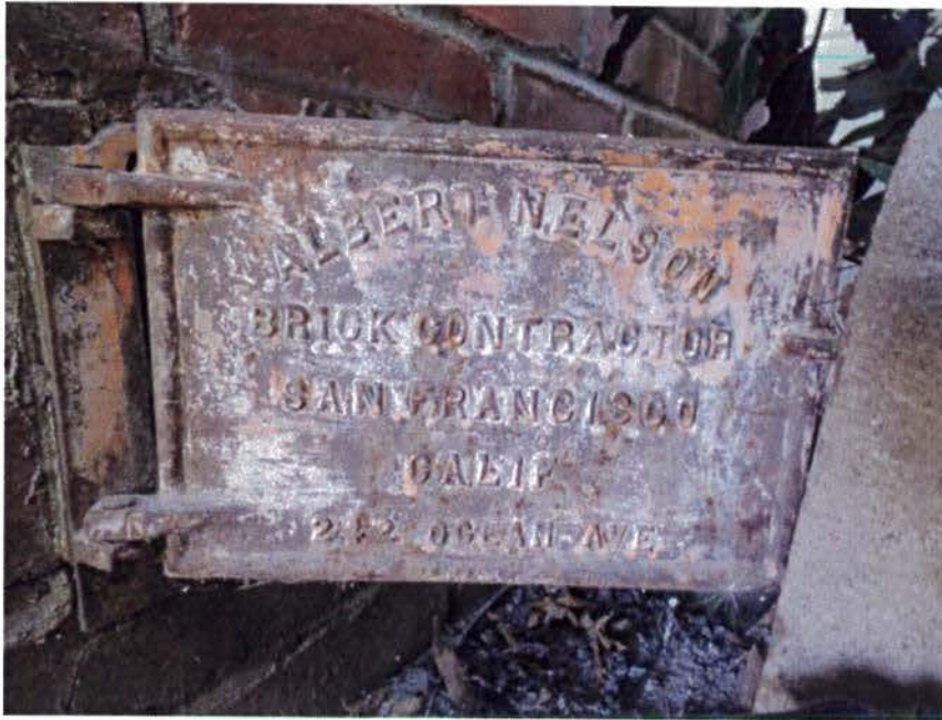
Figure 17. Metal chimney door at west elevation (Garavaglia Architecture, Inc., August 2015)
