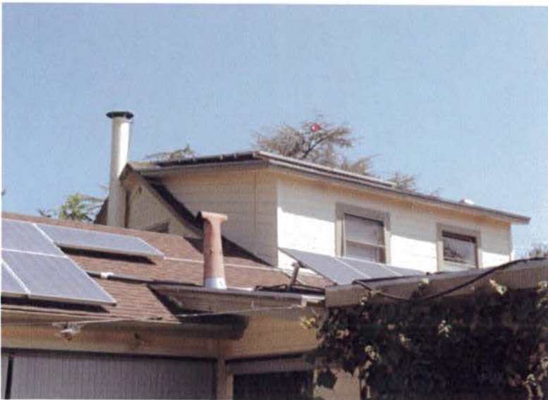
Figure 7. Northeast view of roofline. Note the original second story portion of the home with the Pool House addition to the left and the enclosed porch/kitchen addition to the right (Garavaglia Architecture, Inc., August 2015)
