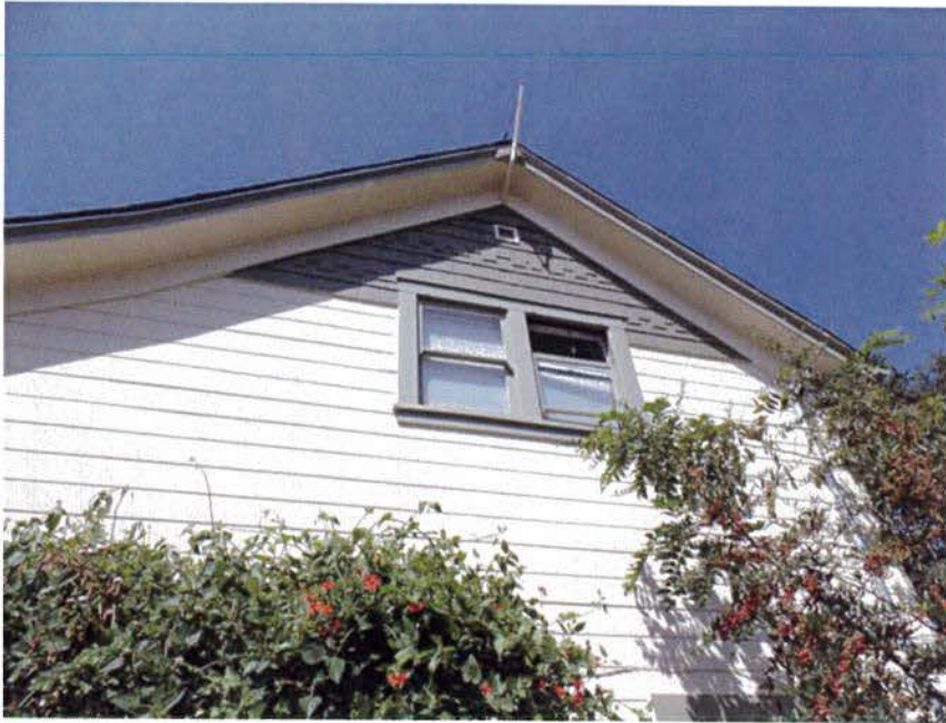
Figure 11. Detail of decorative wood shingles at eastern elevation (Garavaglia Architecture, Inc., August 2015)
