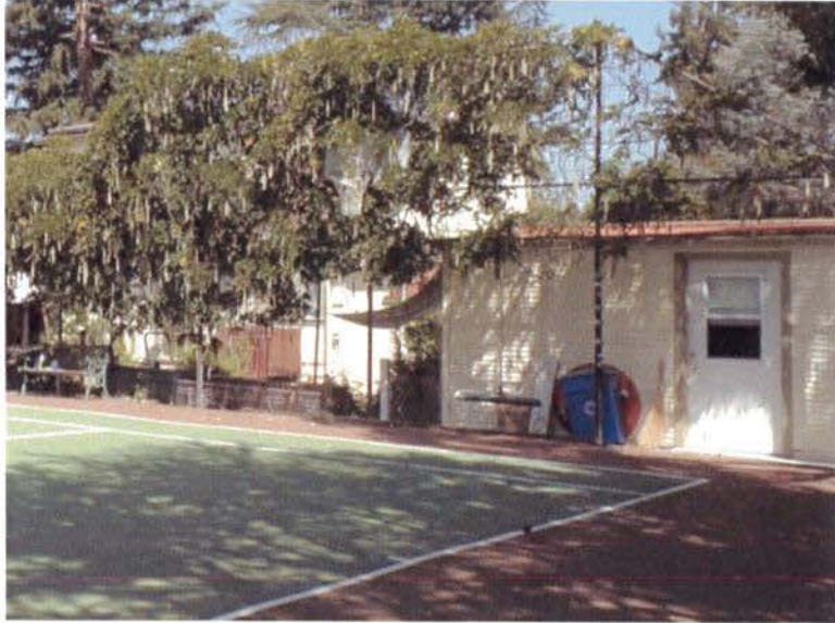
Figure 14. South elevation of Garage addition toward the eastern extent of the property (Garavaglia Architecture, Inc., August 2015)
