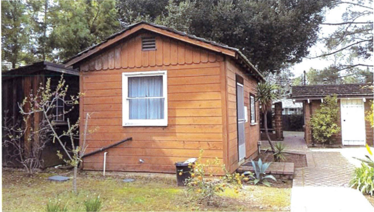
East Elevation, viewed from the northeast
