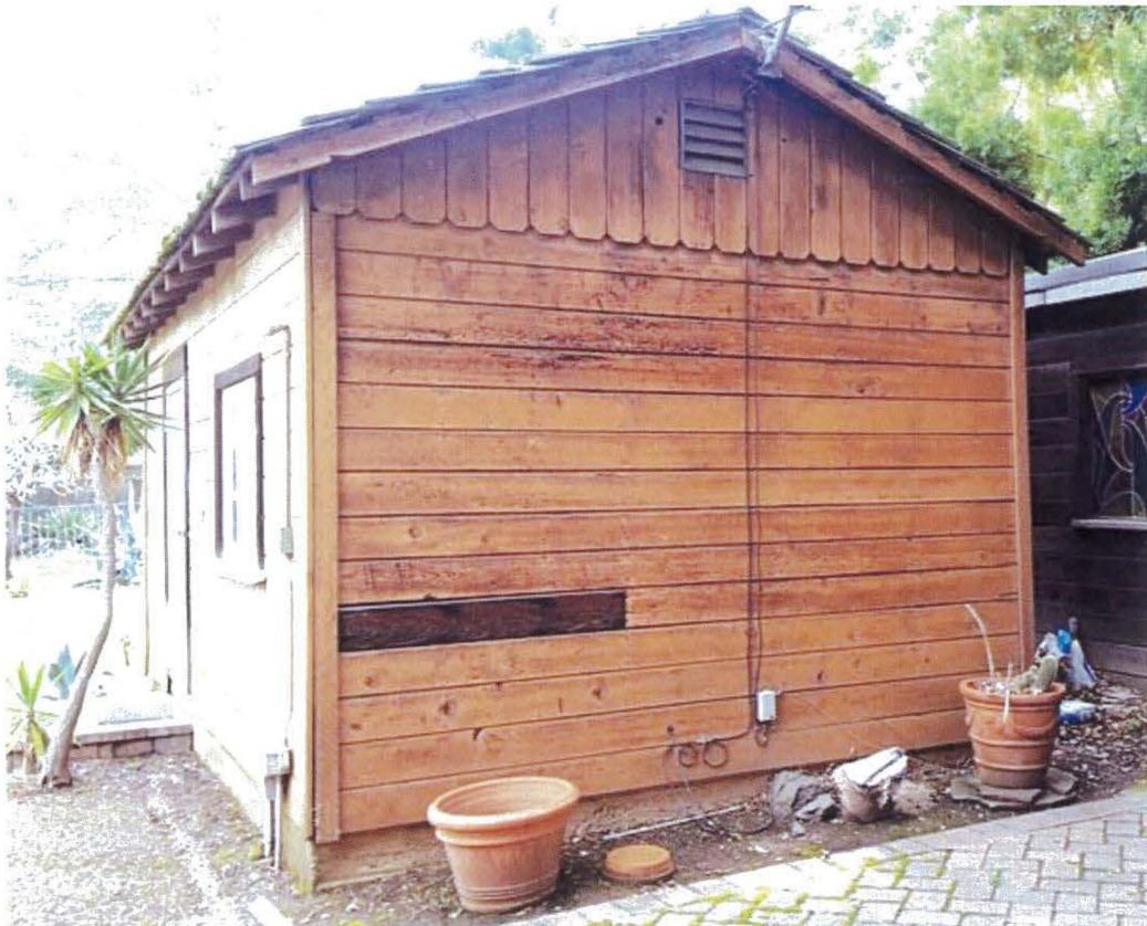
West Elevation, viewed from the west
