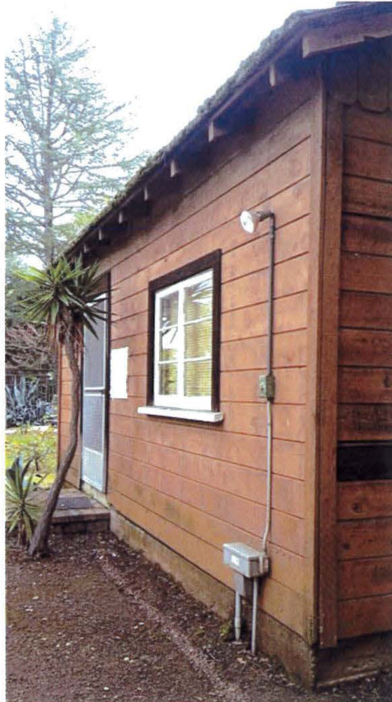
North (Front) Elevation, viewed from the northwest
