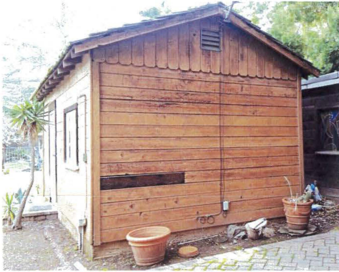
West Elevation, view from the west
