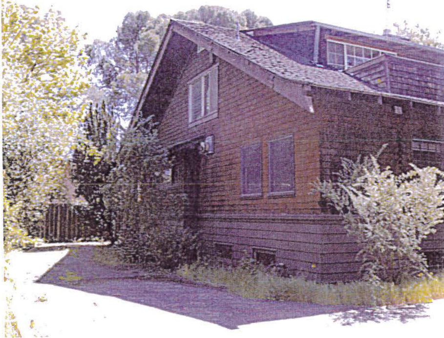
North Elevation, viewed facing southeast.
