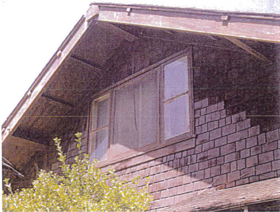
Gable end at south elevation, viewed facing northwest.
