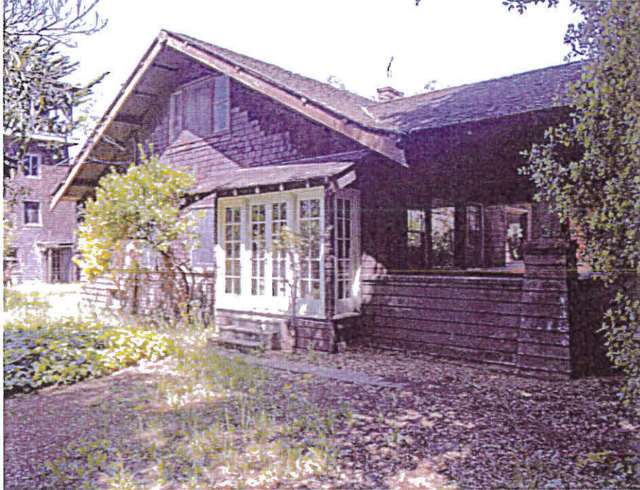
South elevation, viewed facing northwest.
