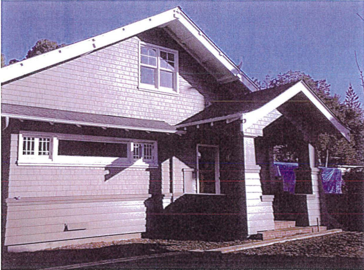
West Side, viewed facing southeast
