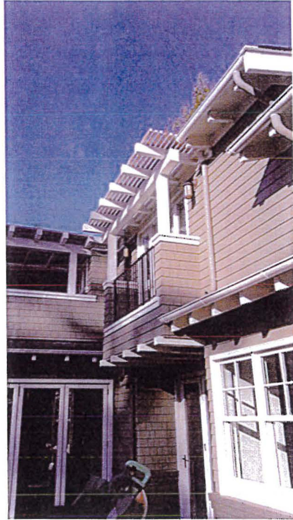
Rear Addition, from the south, showing differentiation of porch overhangs
