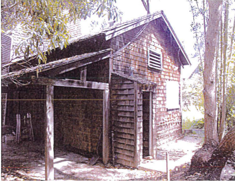
Rear view of addition to tank house, viewed facing northeast.
