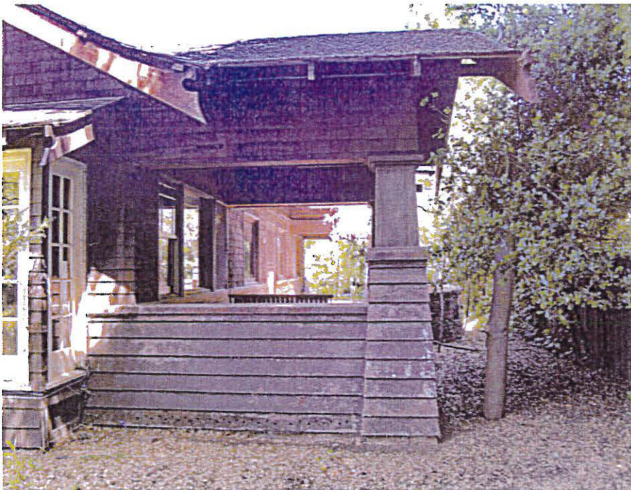
Original front porch, viewed facing north.
