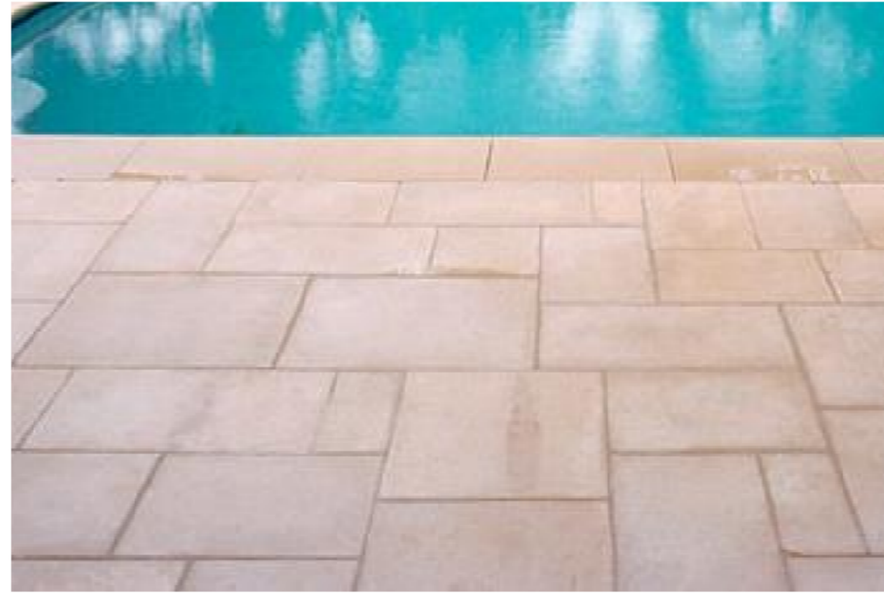
PRECAST CONCRETE PAVING
